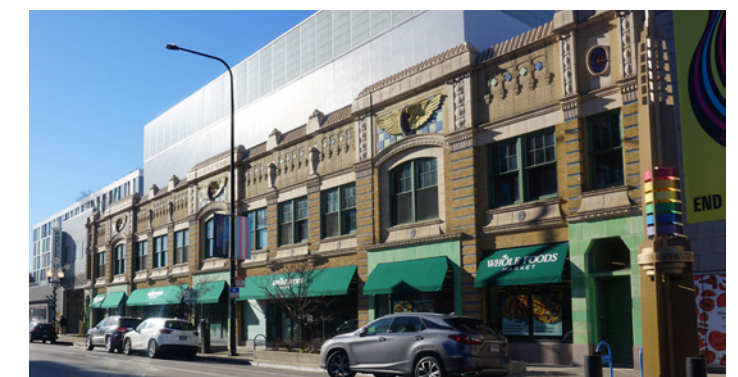
✓ Figure 42. Acceptable example of a facadectomy
