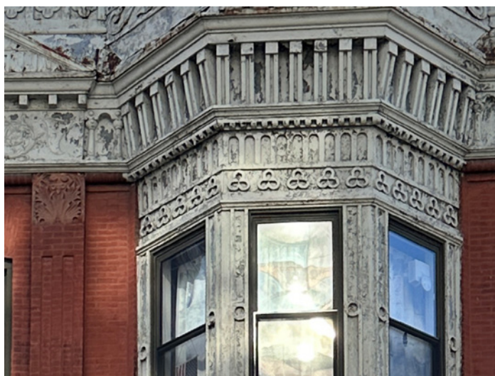
Figure 34. Example of character-defining, historic, architectural metal
