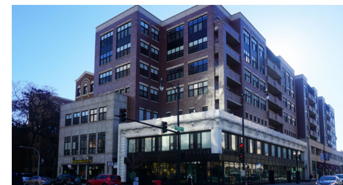
✓ Figure 40. Acceptable example of a facadectomy
