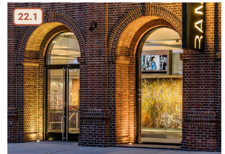
Figure 84. Acceptable example of exterior building lighting
