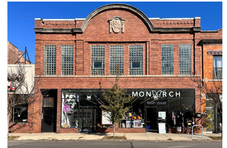
Figure 19. 2875 N Milwaukee Avenue
