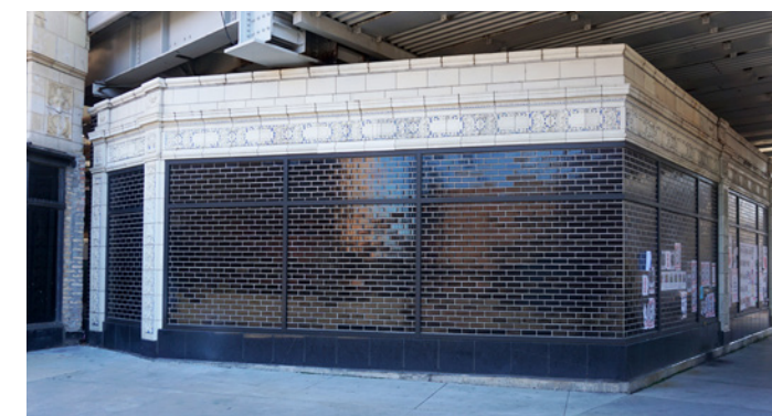
✗ Figure 41. Unacceptable example of a facadectomy as the facade has not been integrated into a new development, but left as an unoccupiable portion of a building and the storefront infilled with brick and a fake storefront frame
