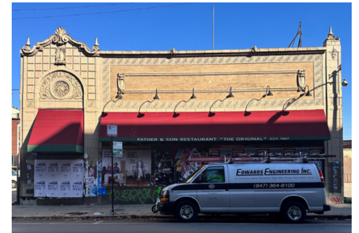
Figure 20. 2475 N Milwaukee Avenue
