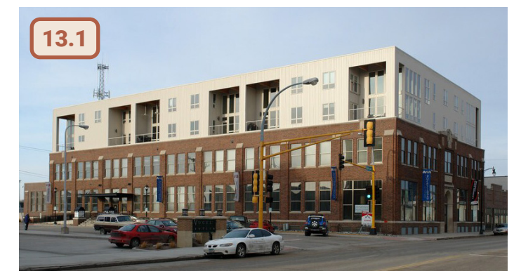
✗ Figure 60. Unacceptable example of a design for an addition to an existing building due to incompatible materials and design of fenestration/recesses (Loopnet)
