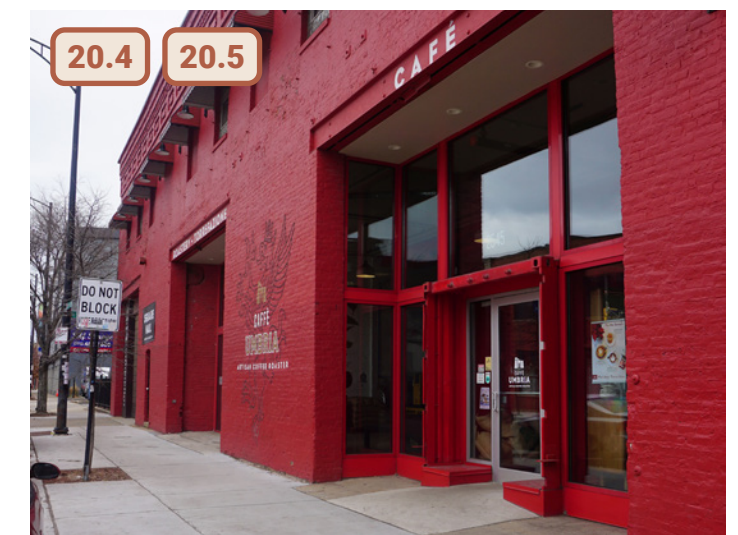
✓ Figure 77. Acceptable example of deeply recessed storefront and entry
