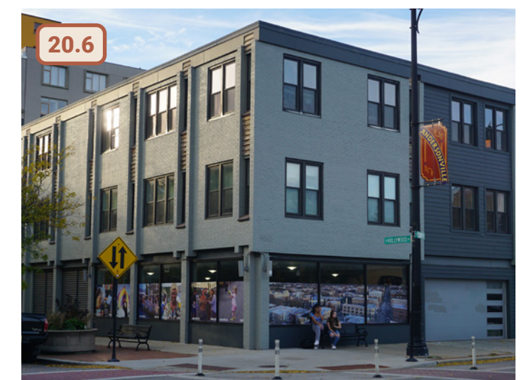
✗ Figure 78. Unacceptable example of fake storefront in new construction designed to screen ground floor parking
