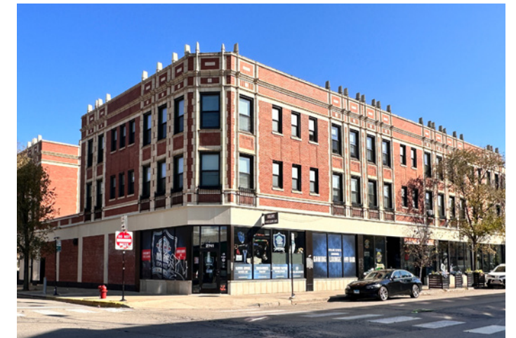
Figure 118. 2741 N Milwaukee Avenue
