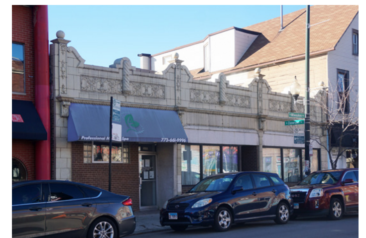
Figure 21. 2832 N Milwaukee Avenue
