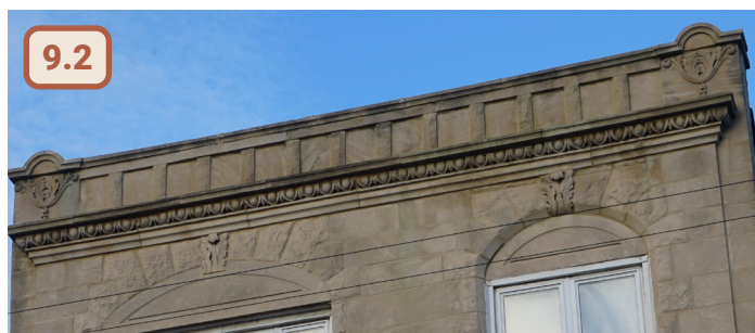
Figure 52. Examples of existing cornices in the district
