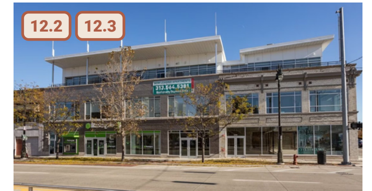
✗ Figure 59. Unacceptable example of an addition as the addition has a projecting roofline that does not minimize its visibility (Apartments.com)
