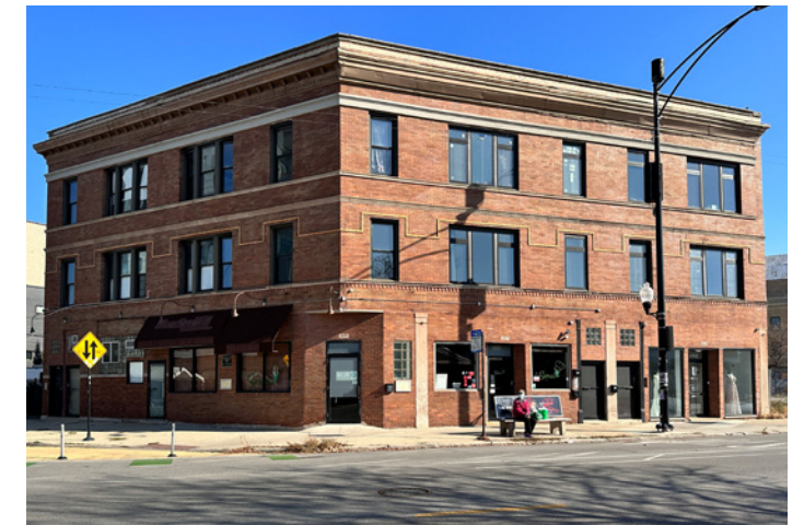
Figure 119. 2171 N Milwaukee Avenue
