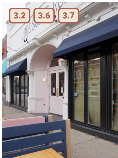
✓ Figure 38. Acceptable example of a new storefront that retained character-defining features of the original storefront
