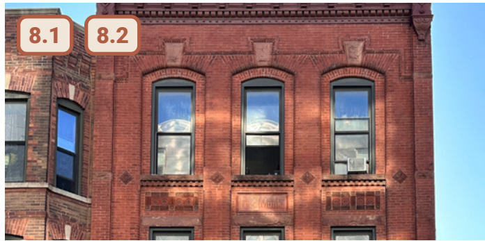
✓ Figure 48. Acceptable example of new windows in preserved masonry openings
