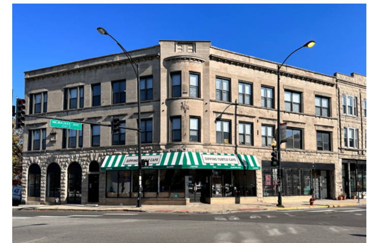
Figure 120. 2959 N Milwaukee Avenue
