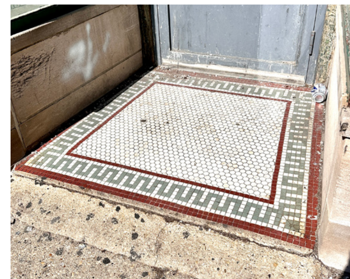
Figure 183. Acceptable example of historic storefront flooring
