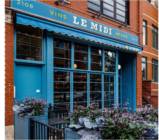
Figure 55. Facades, awnings, and window signage (Source: Le Midi Wine)
