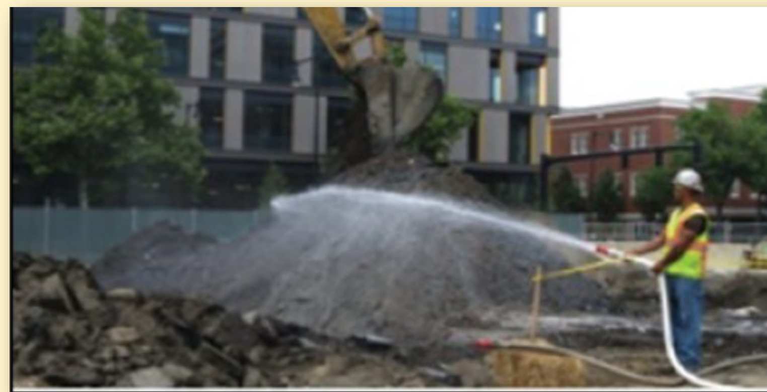
Erosion Prevention - Tackifier
