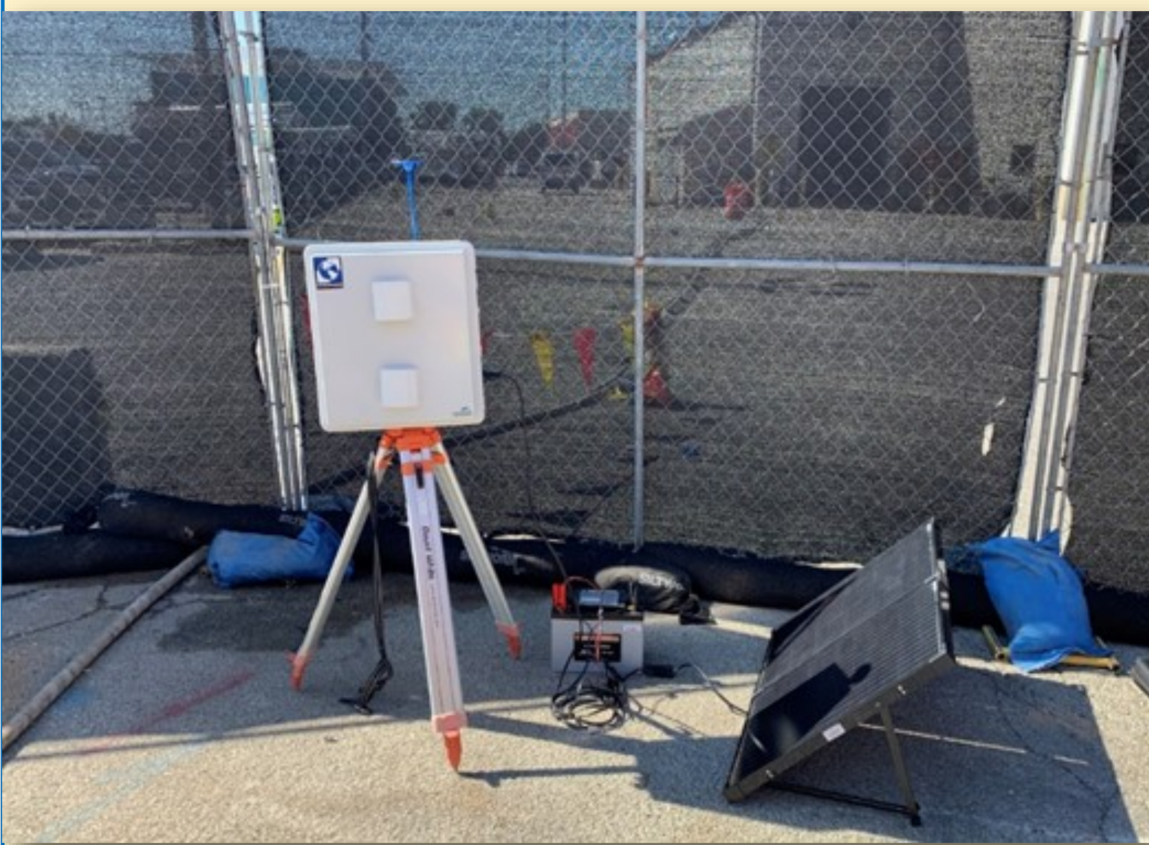
Typical Air Monitoring Station
