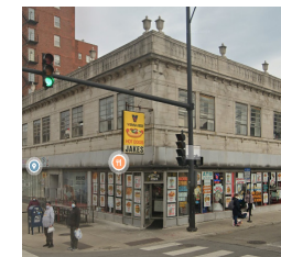
4401 N. Sheridan Rd. (photo from Google Street View)
