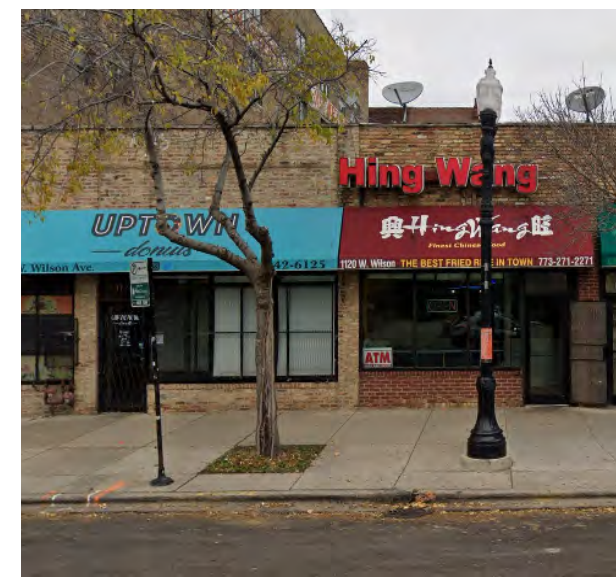
1118 W. Wilson Ave. (photo from Google Street View)
