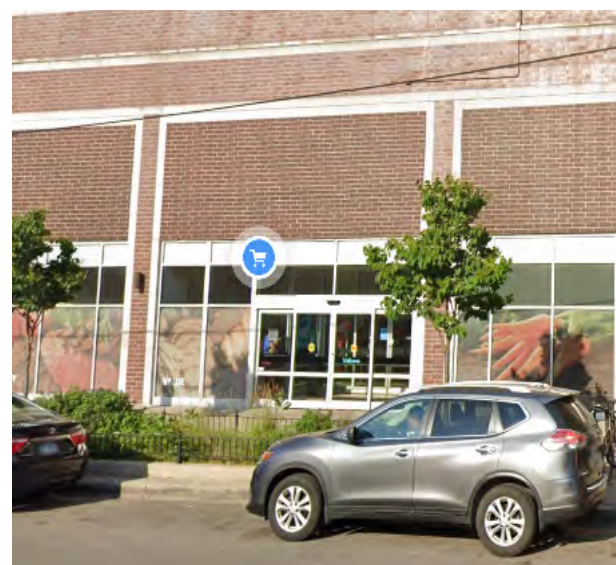
6221 N. Broadway (photo from Google Street View)
