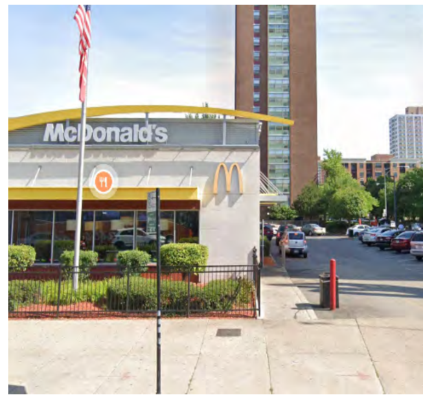
1004 W. Wilson Ave. (photo from Google Street View)
