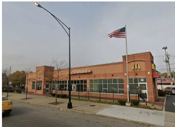
Street view facing North
