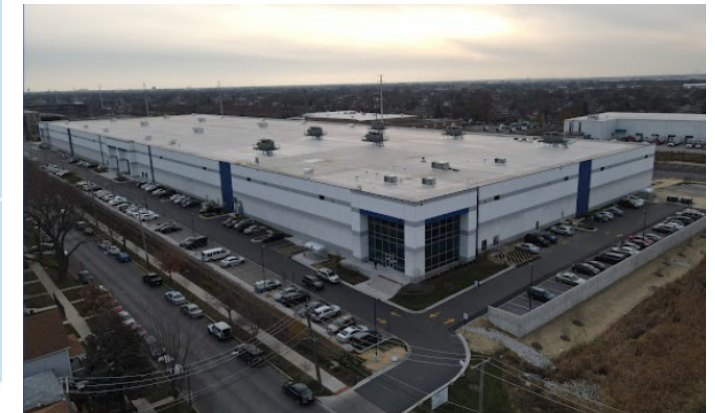
B Amazon | 3507 W 51st St 316,550 SF • Construido 2019
