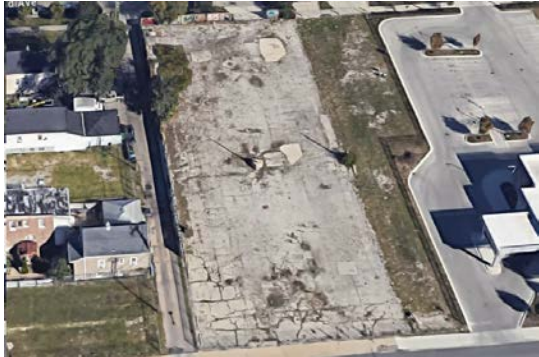
28 Vacant land parcels with minor improvement
