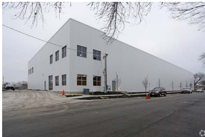
C 5115 S Millard Avenue 42,000 SF • Cold Storage • 2016 • Moesle Meats
