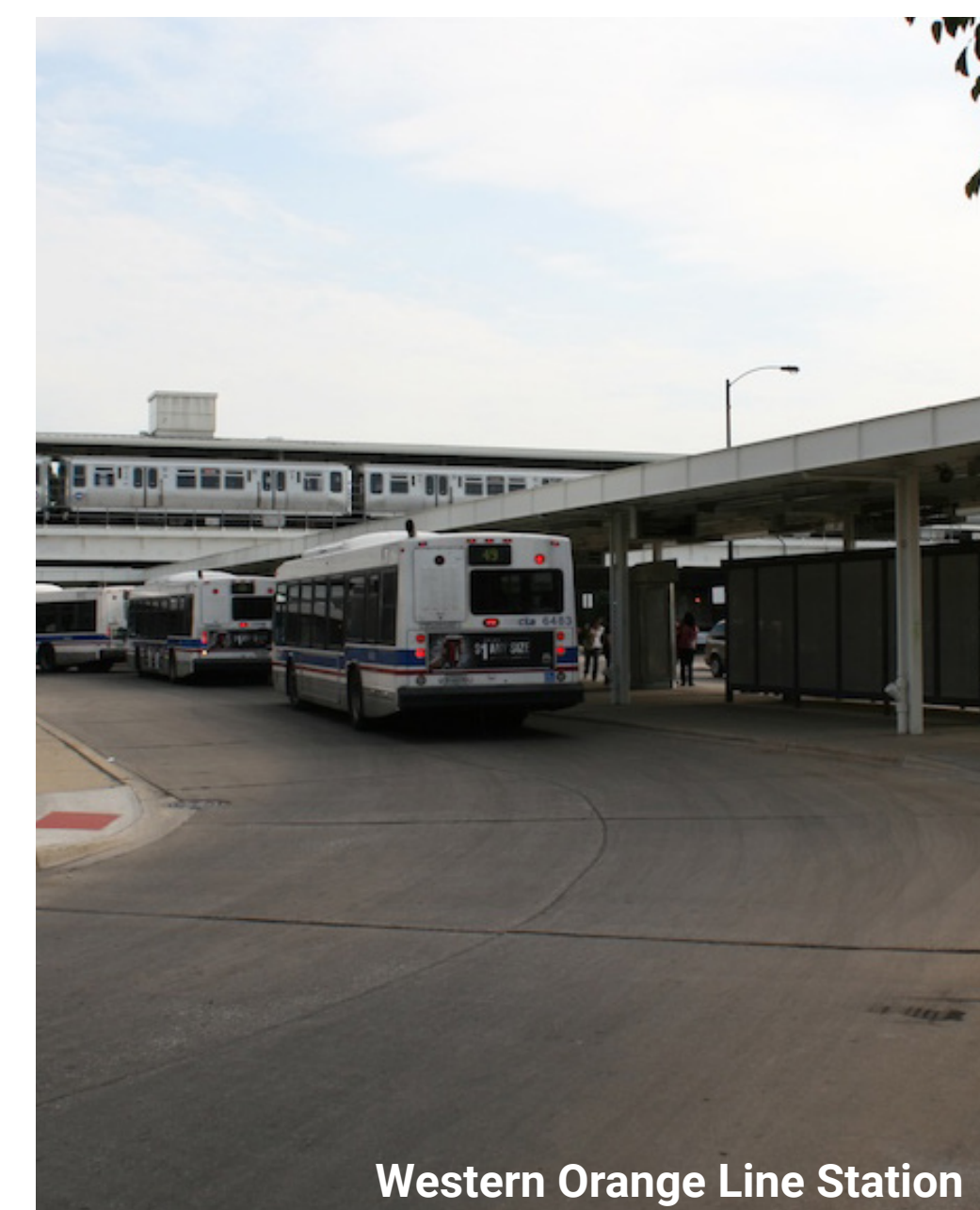
Western Orange Line Station
