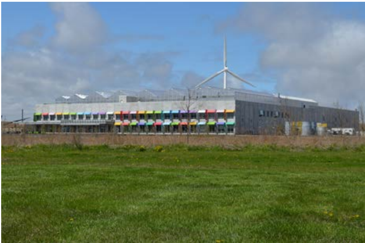
Method Factory, Calumet Industrial Corridor
