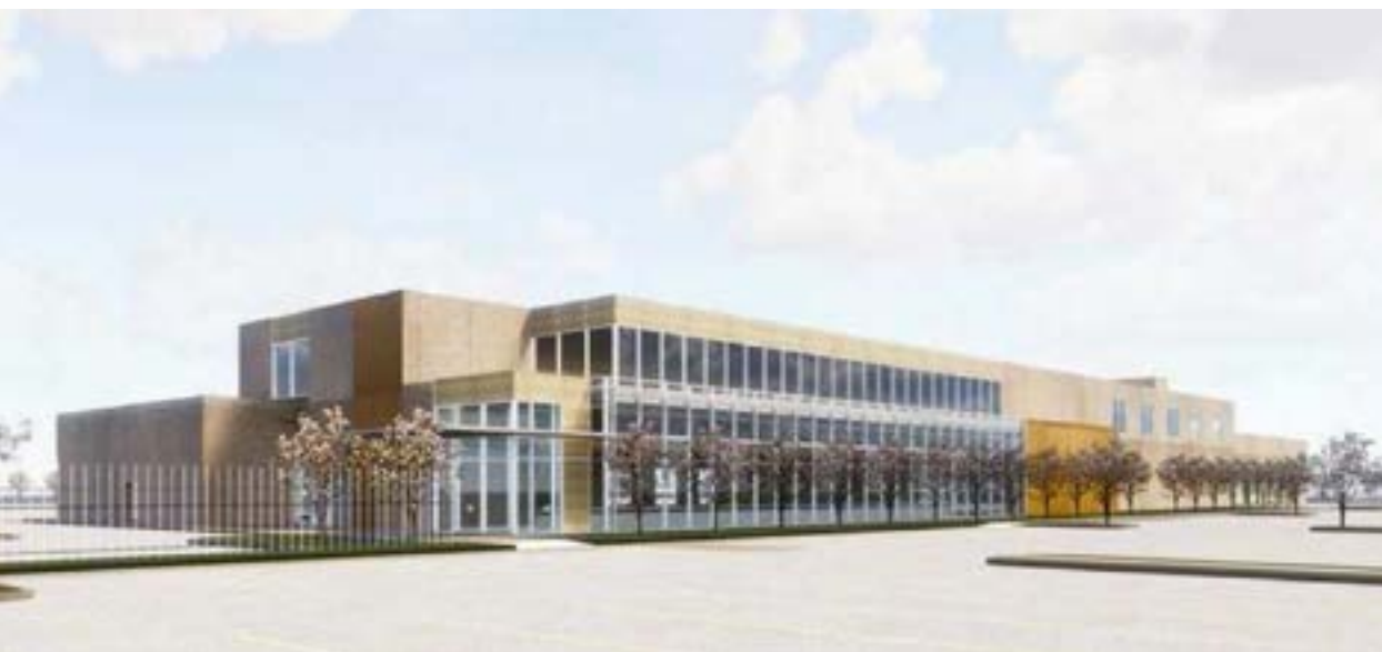
Peoples Gas Facility
