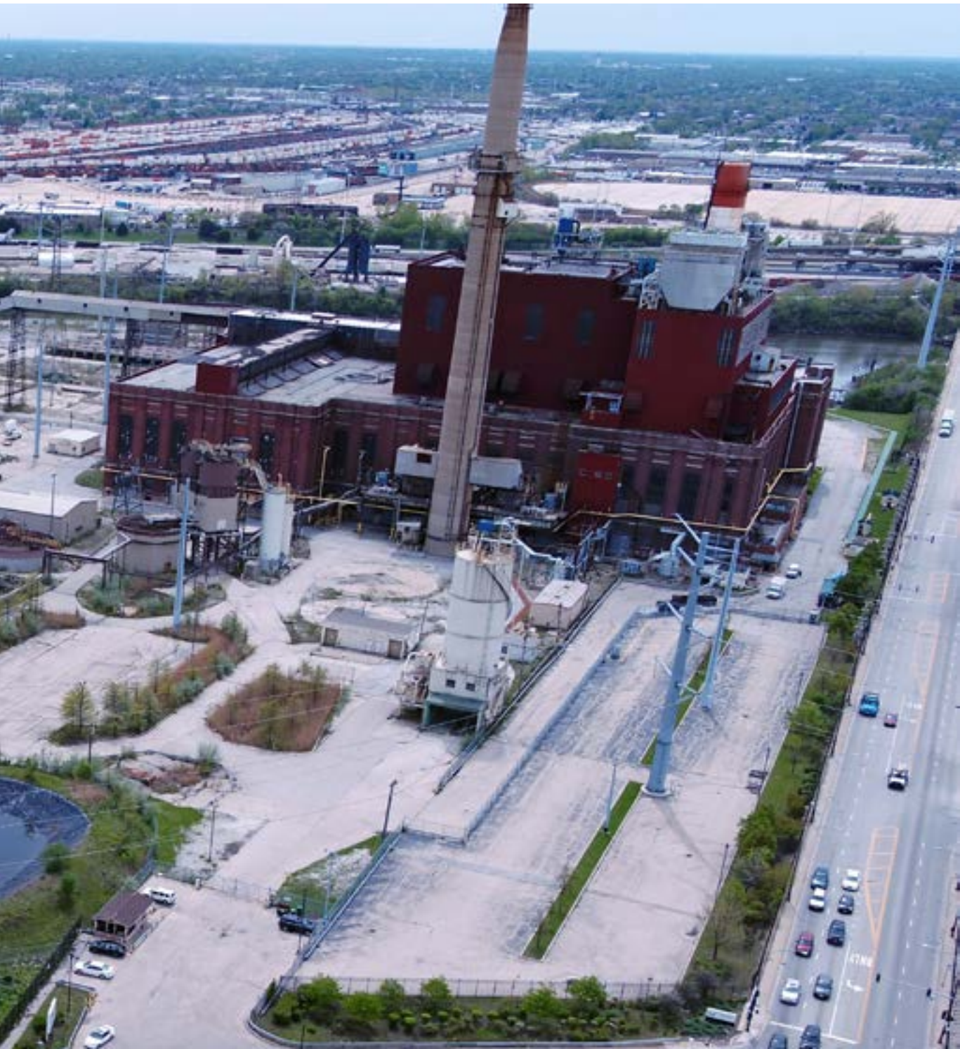
Crawford Power Generation Plant, Pulaski Road & 35th Street
