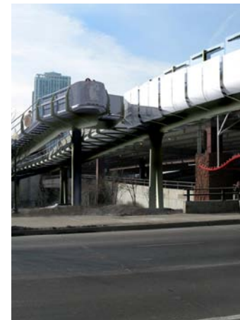
Image 3-27: The new bridge will separate bicycle and pedestrian traffic from the existing street crossing.
