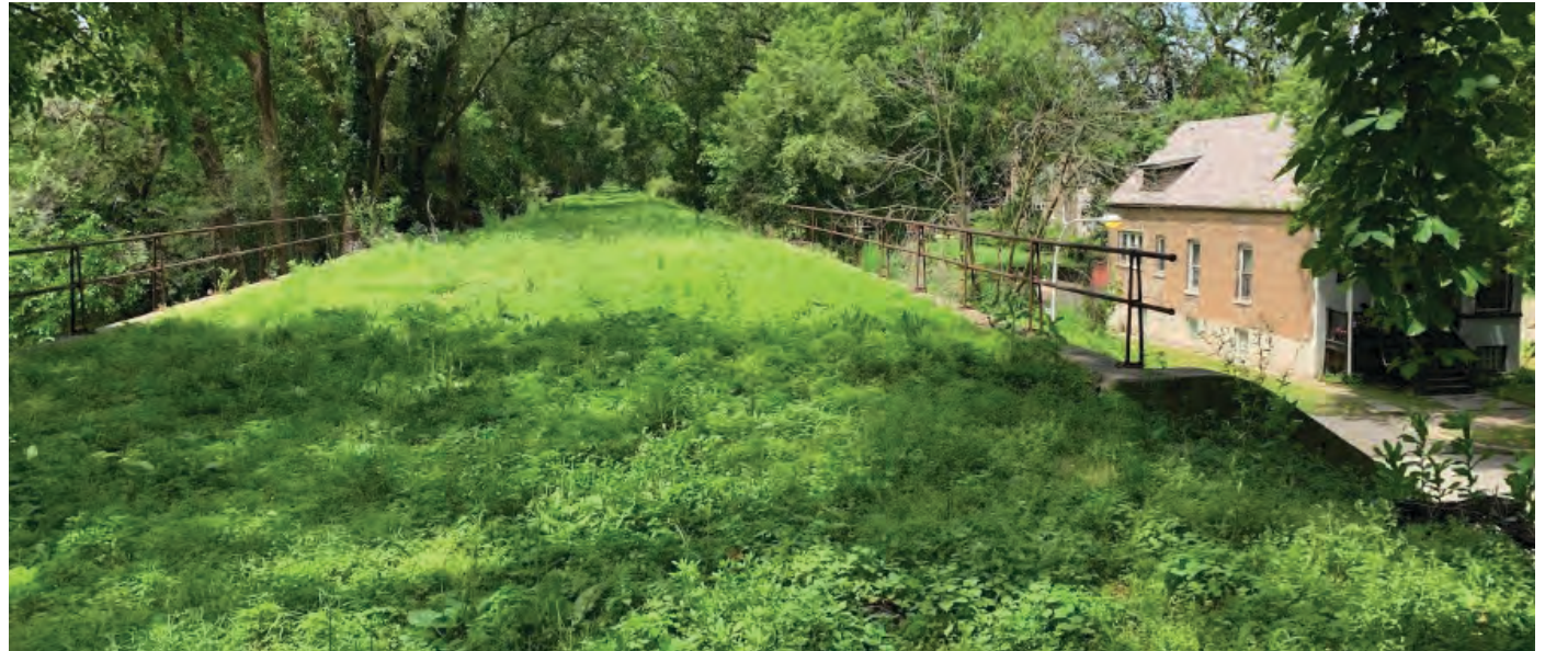
Existing elevated trail.
