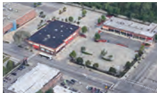
Former CVS Pharmacy Site
