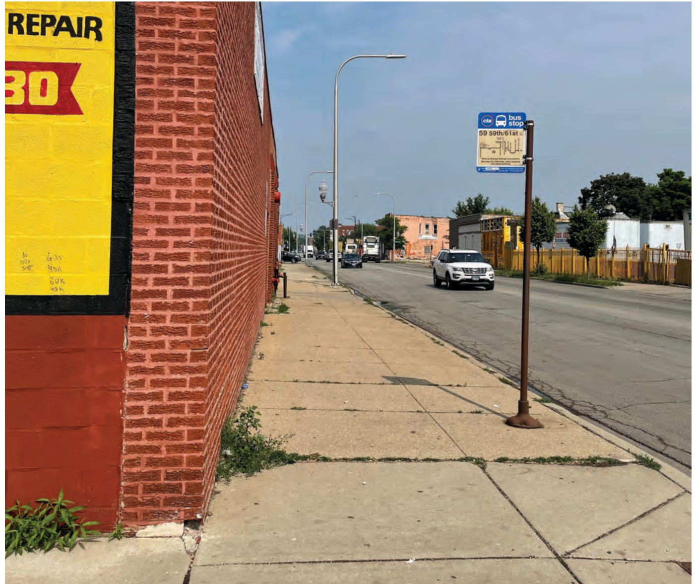
Existing 59th Street streetscape
