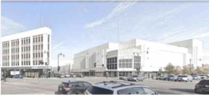
VIEW OF EXISTING SEARS BUILDING
