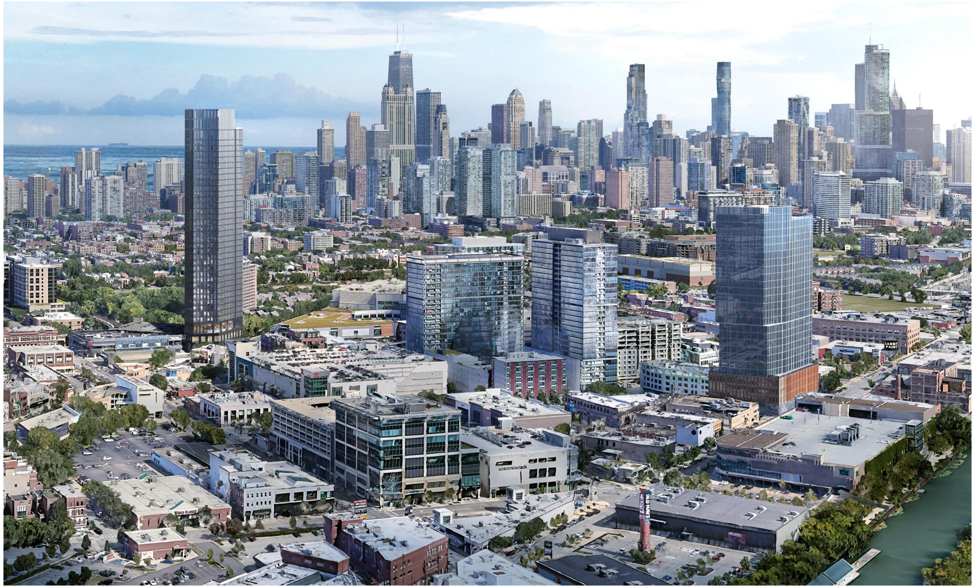
OVERALL BUILDING – VIEW FROM NORTHWEST
