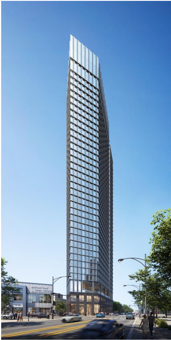
OVERALL BUILDING – VIEW FROM NORTHWEST
