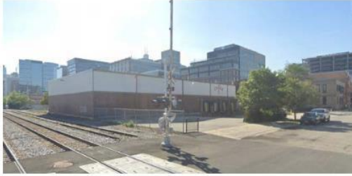
North West Corner
