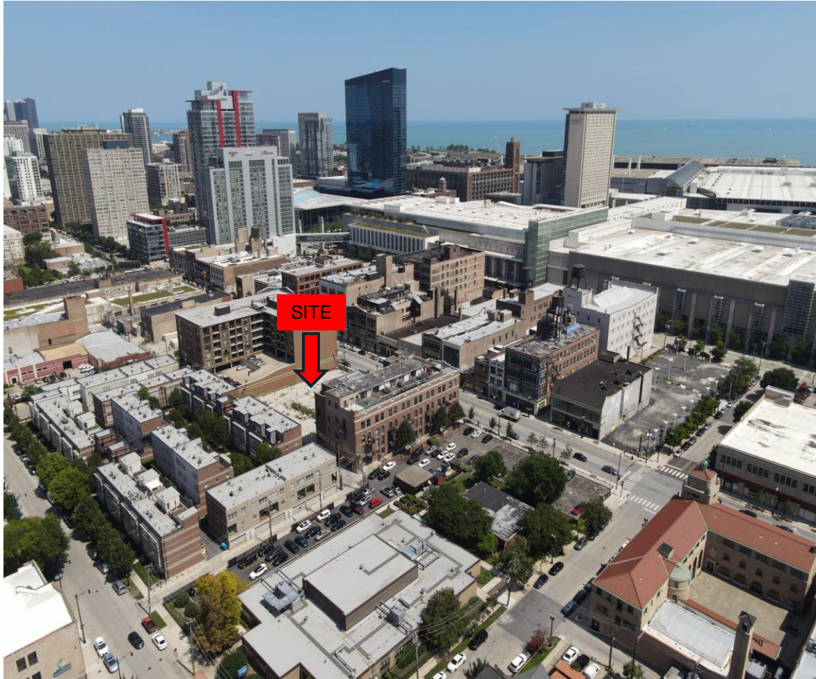
Aerial from South West Looking North East
