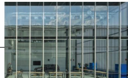
Curtain Wall Glazing
