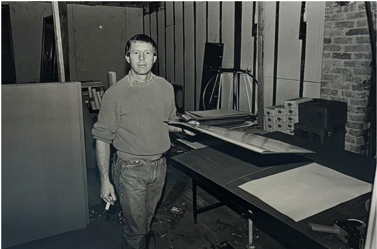
Above: Dannie Flesher building out the rear addition.
