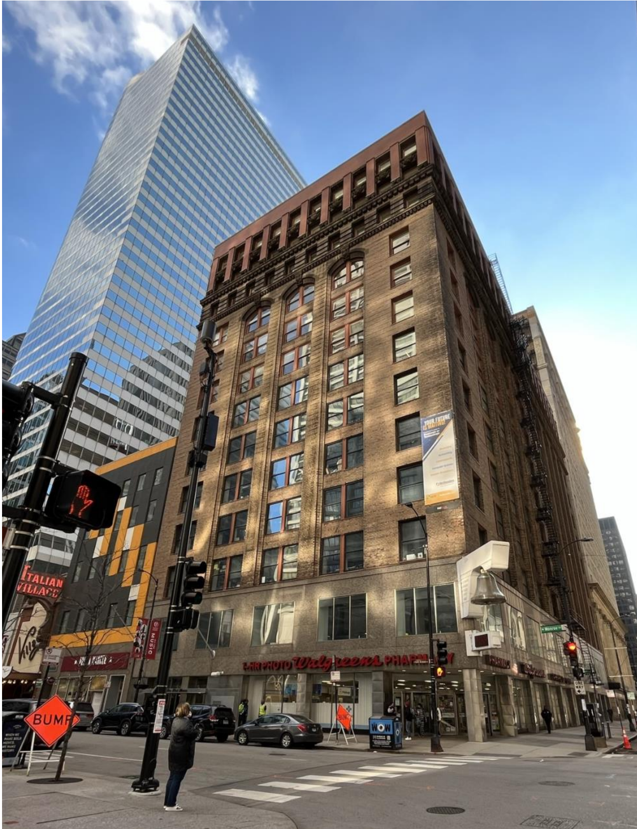
North elevation and west elevation of the Rector Building, looking southeast at the intersection of Clark and Monroe Street.
