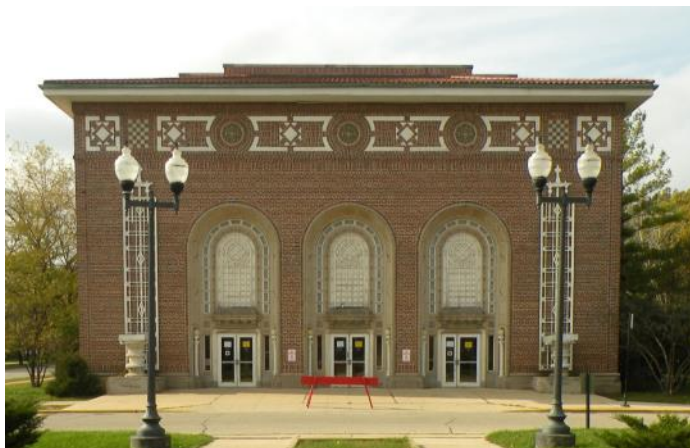
Bottom left: Hunt's 1919 design for the Auditorium Building at the Chicago Municipal Tuberculosis Sanitarium combined Italian Renaissance Revival and Prairie School elements. Source: Municipal Tuberculosis Sanitarium Complex, Chicago Landmark Designation Report.
