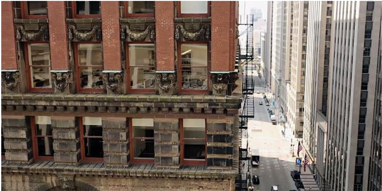
Detail of the terra-cotta ornamentation at the upper stories of the Rector Building. (Photograph by R2).
