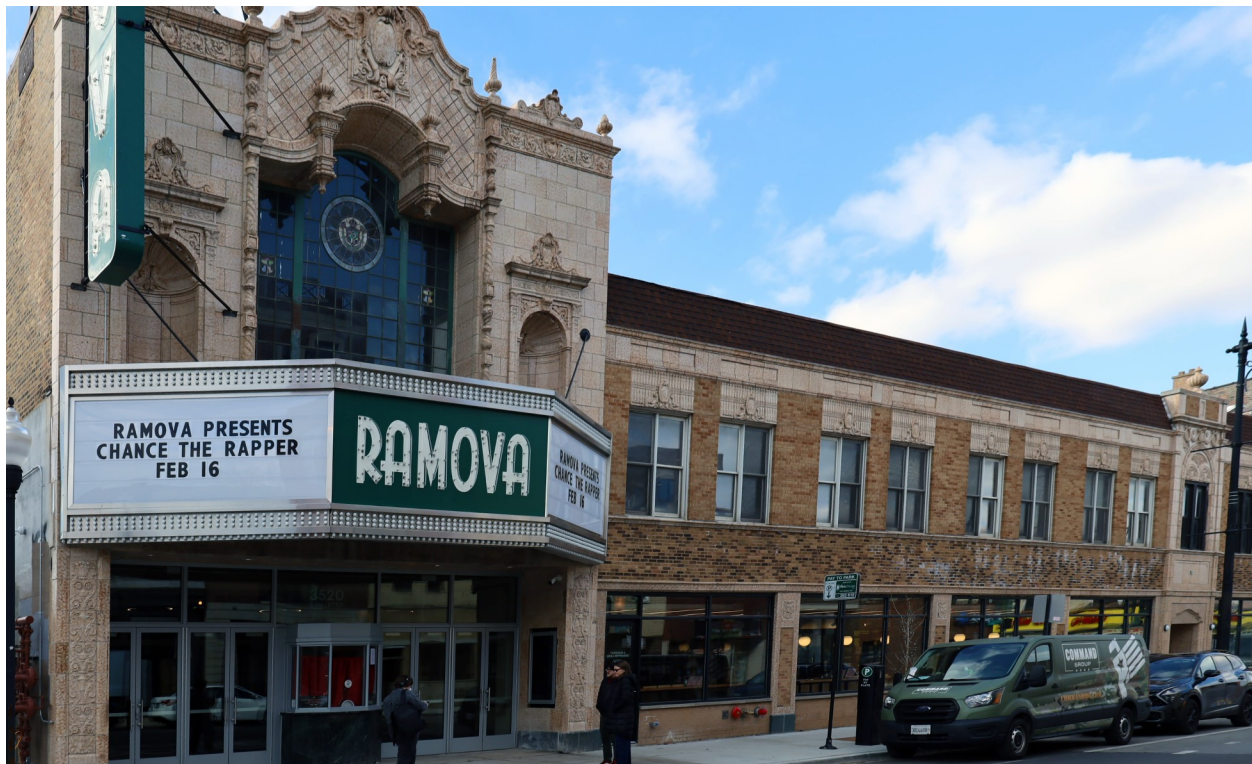
Current view of the Ramova Theater looking north on South Halsted Street. The theater's façade at left is from 1929. The commercial wing at right was built in 1912, then a story and a new façade were added in 1929 to compliment the theater.
