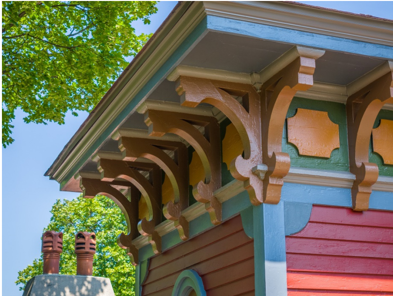
Left: Bracketed cornice and decorative frieze band under the eaves of the tower's hip roof.
