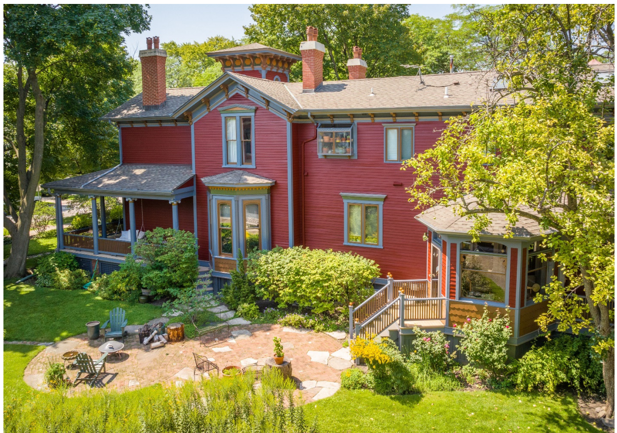
Top Photo: South Elevation, wood trim detailing Bottom Photo: East Elevation, including a later 1-story rear addition. The farmhouse's original rear wall was immediately south of the pictured addition. Source: Troy Walsh, Drone Media Chicago (2023)
