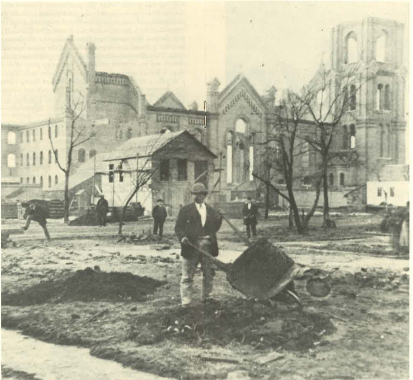
This photograph, taken shortly after the Chicago Fire of 1871, shows the ruins of St. Michael's Church. The double walls on the south, east, and west ends of the church withstood the fire. Within one year and three days after the fire, the industrious parishioners of St. Michael's Church rebuilt the damaged structure. Chicago cottages like the one pictured in the center of the photograph dotted the area within days after the fire and were sometimes referred to as "relief shanties." (Courtesy of Chicago Historical Society)
