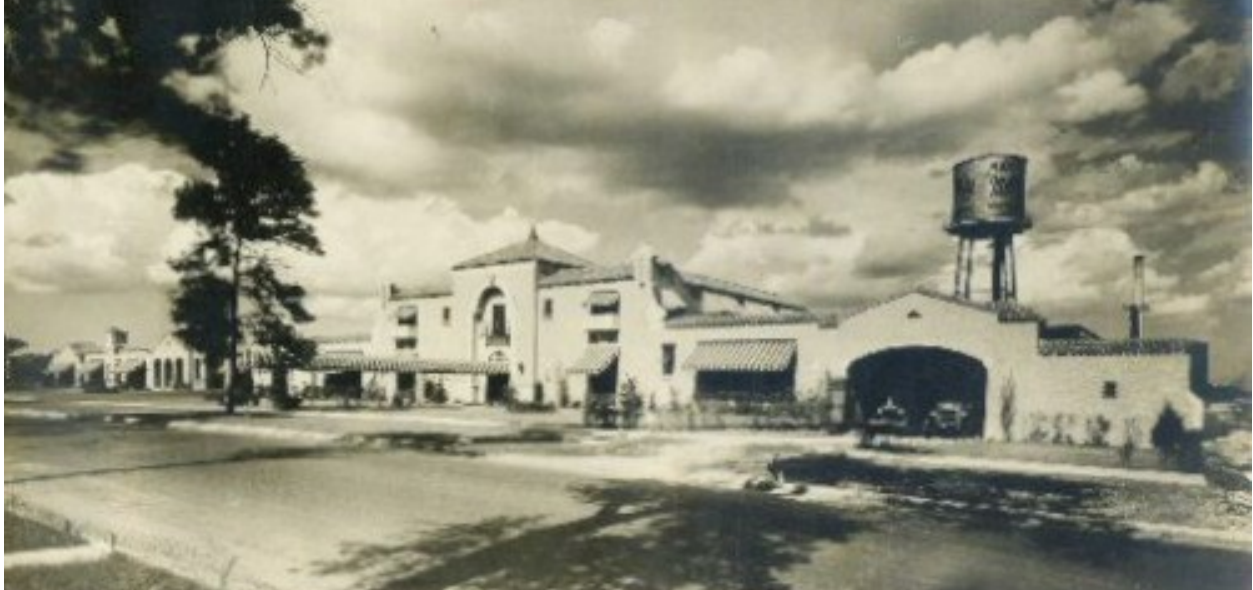
The Mars Candy Factory, sometime between 1929-1947. The south wing incorporated a large arched opening for truck access from Oak Park Avenue, later infilled. (Source: Calumet 412)
