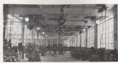
Interior of Dominion Steel Products Co. building, showing well-lighted machine room.
