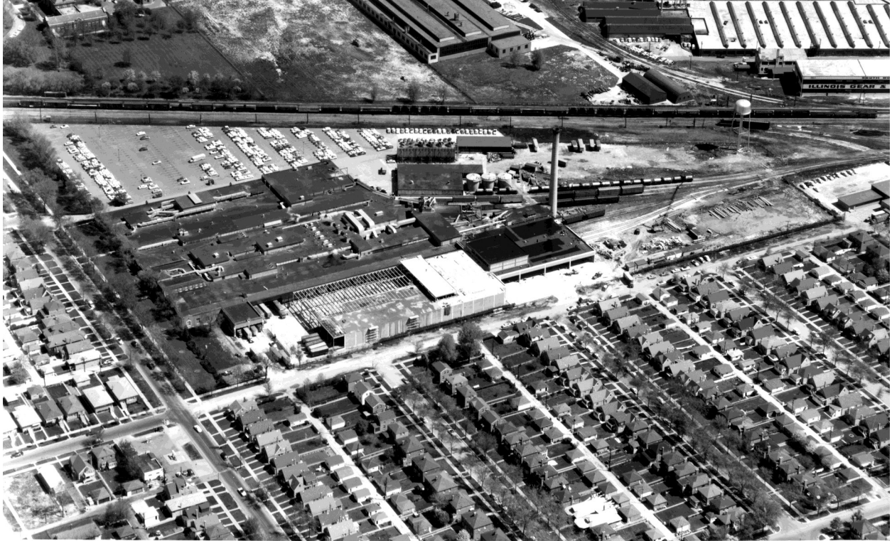
This aerial photo, taken May 7, 1958, includes the Mars Candy Factory and surrounding area. The 1960 addition has not yet been built. (Photo provided by Tom Drebenstedt. Source: The Milwaukee Road Collection, John W. Barriger III National Railway Library, posted on flickr.com.)
