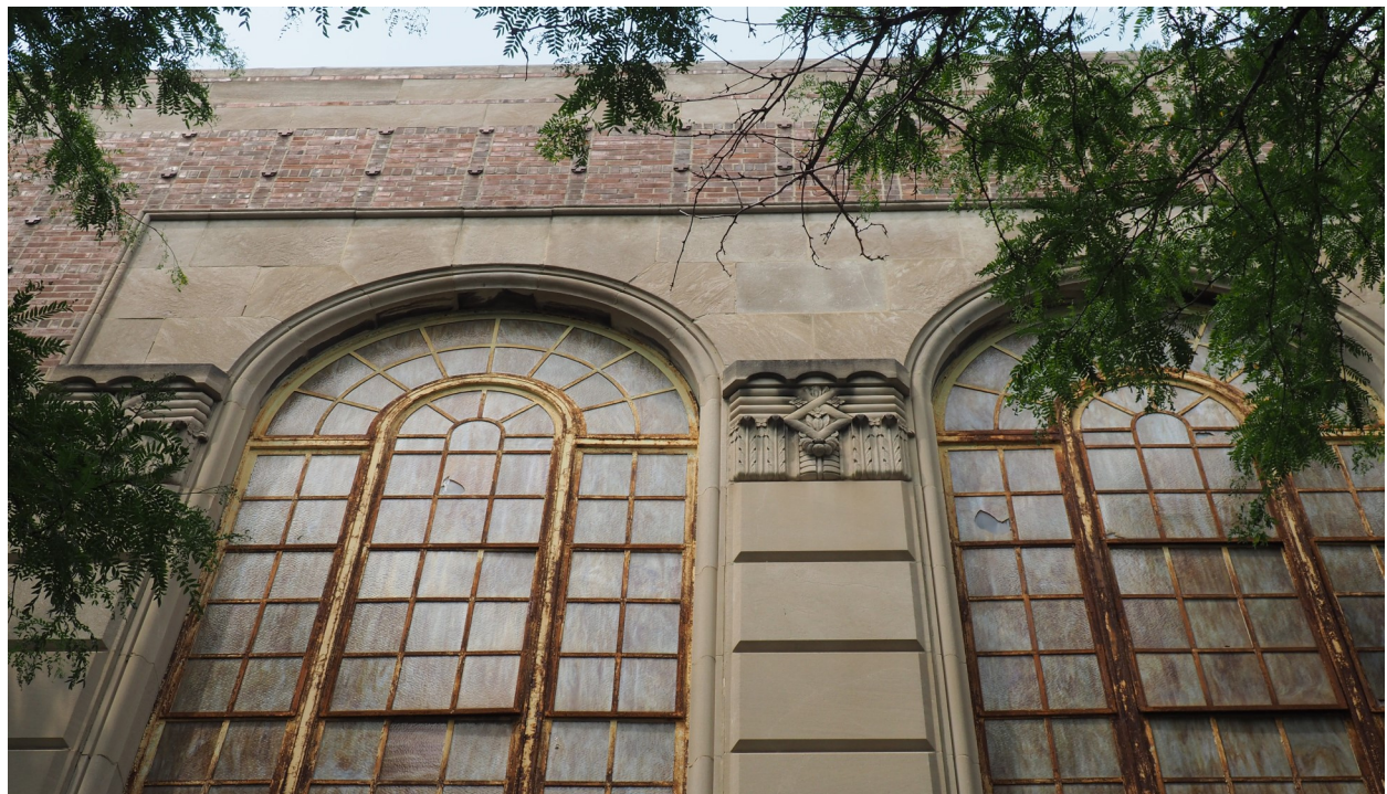
The south (Fulton Street) façade is characterized by a monumental three-story tall limestone arcade which corresponds to the auditorium on the interior as depicted above. The arcade is framed by compounded mouldings and flanked by limestone capitals adorned with stylized classical and geometric motifs as pictured below.
