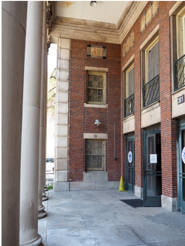
On the interior of the portico, the building expresses refined and simplified Neoclassical details including limestone quoins and bronze Juliette balconies as pictured to the left and coffered panels and lamb's tongue and compounded mouldings rendered in carved limestone.
