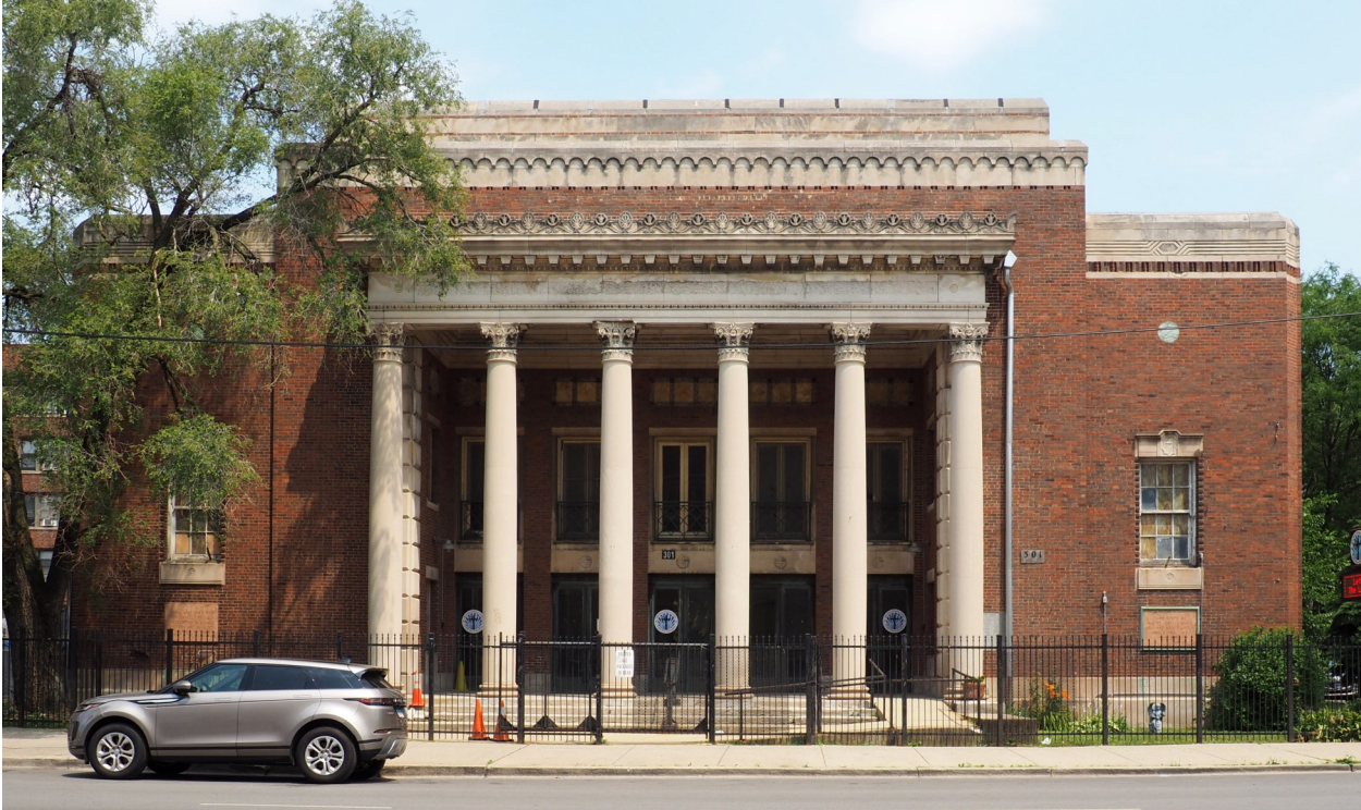
The front (Central Avenue) façade is defined by a striking Neoclassical portico framed by six colossal Corinthian columns which support an intricately carved entablature. Above the portico the façade displays stylized limestone architectural detailing along the cornice line and parapet wall inspired by the Art Deco style.
