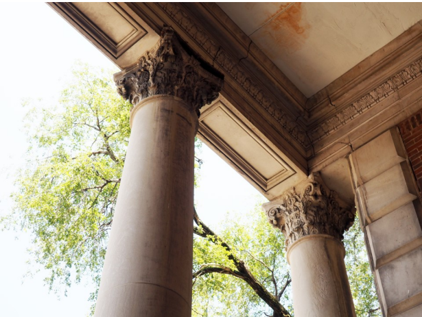
On the interior of the portico, the building expresses refined and simplified Neoclassical details including limestone quoins and bronze Juliette balconies as pictured to the left and coffered panels and lamb's tongue and compounded mouldings rendered in carved limestone.
