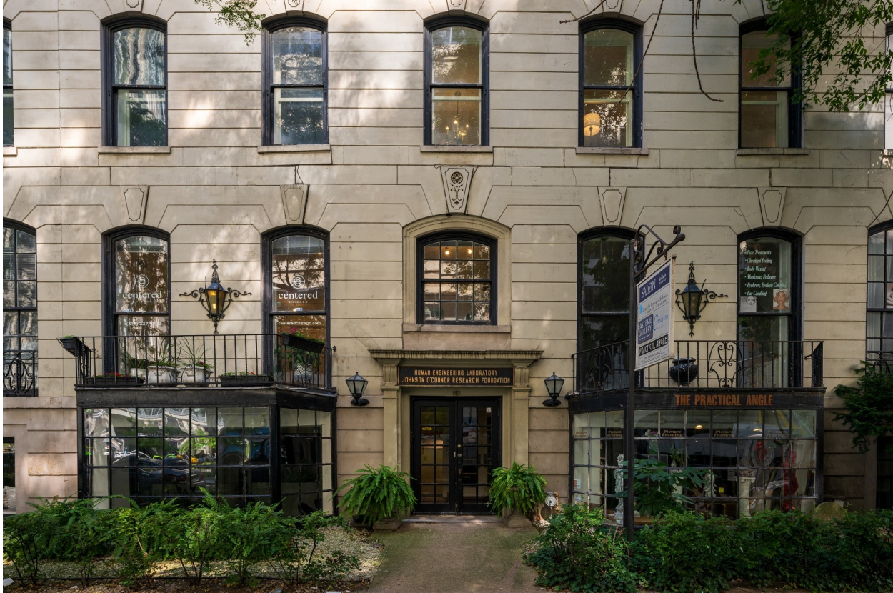
In the 1920s transformation of the Erie Street Row, bay windows topped with balconies were added and the raised entrances to each townhouse were consolidated to a single entrance at grade.
