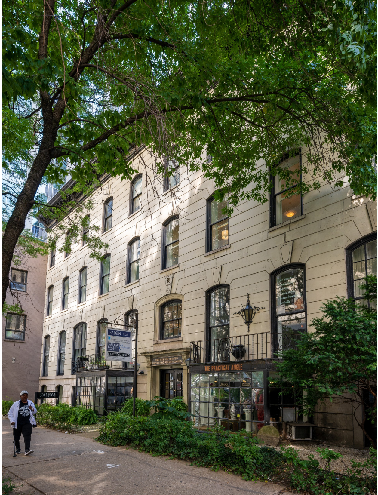
The front façade of the Erie Street Row features rusticated horizontal joints, segmented arch windows with projecting keystones and a pressed metal cornice, all defining features of the Italianate style of architecture.
