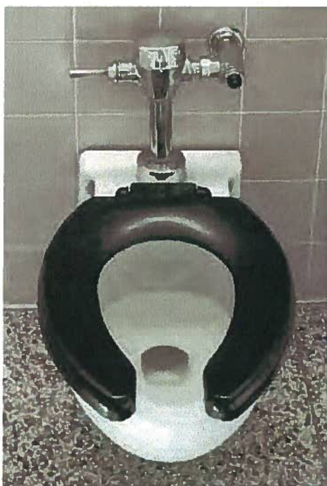
Flushometer-valve toilet
