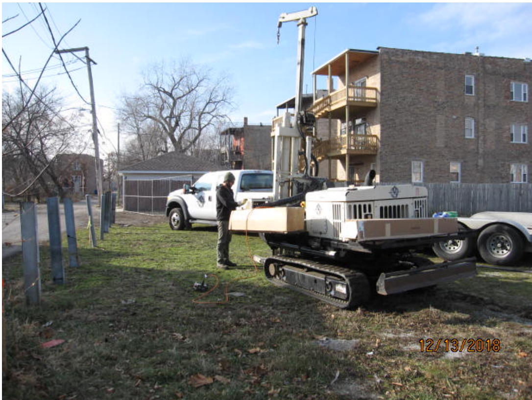
Photo 12: Advancement of soil boring SB-10.
