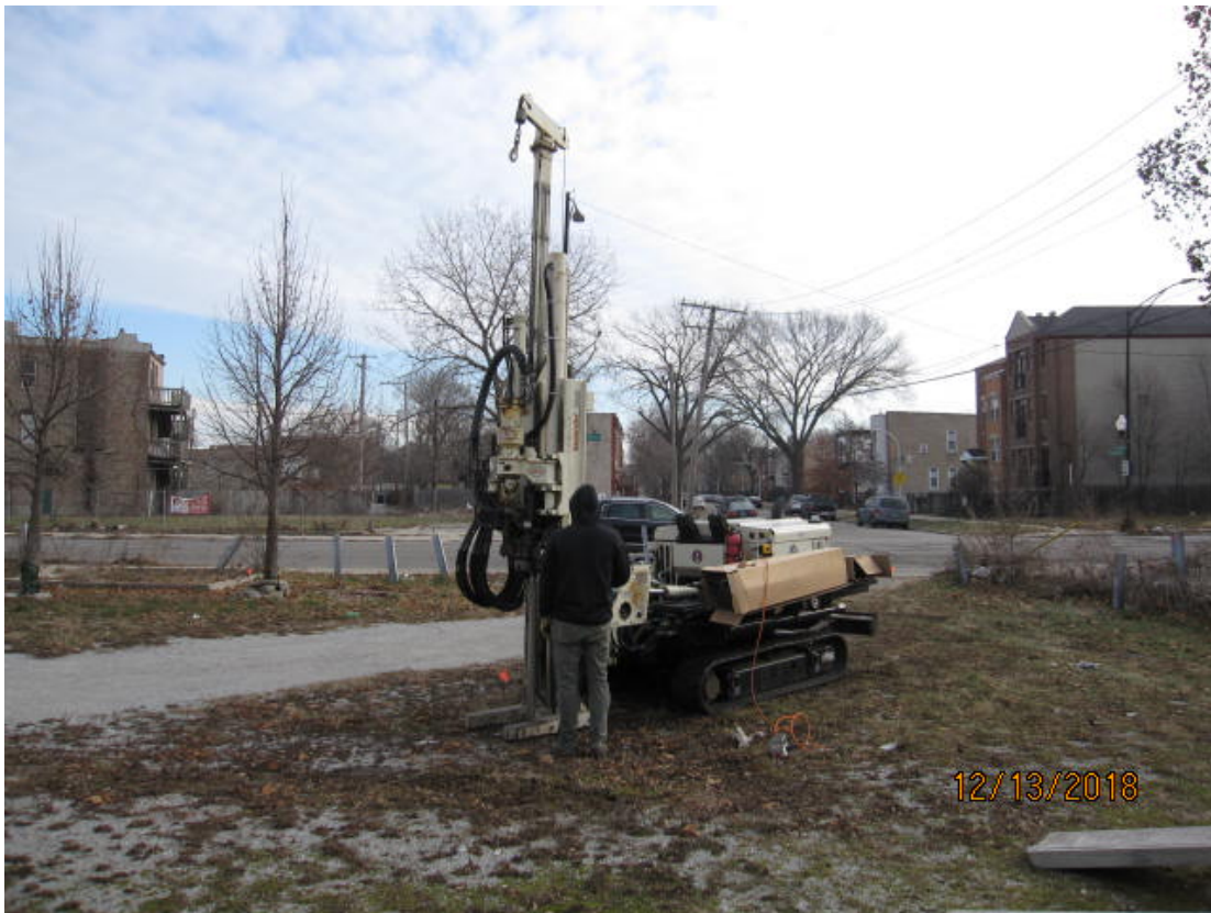
Photo 7: Advancement of soil boring SB-5.
