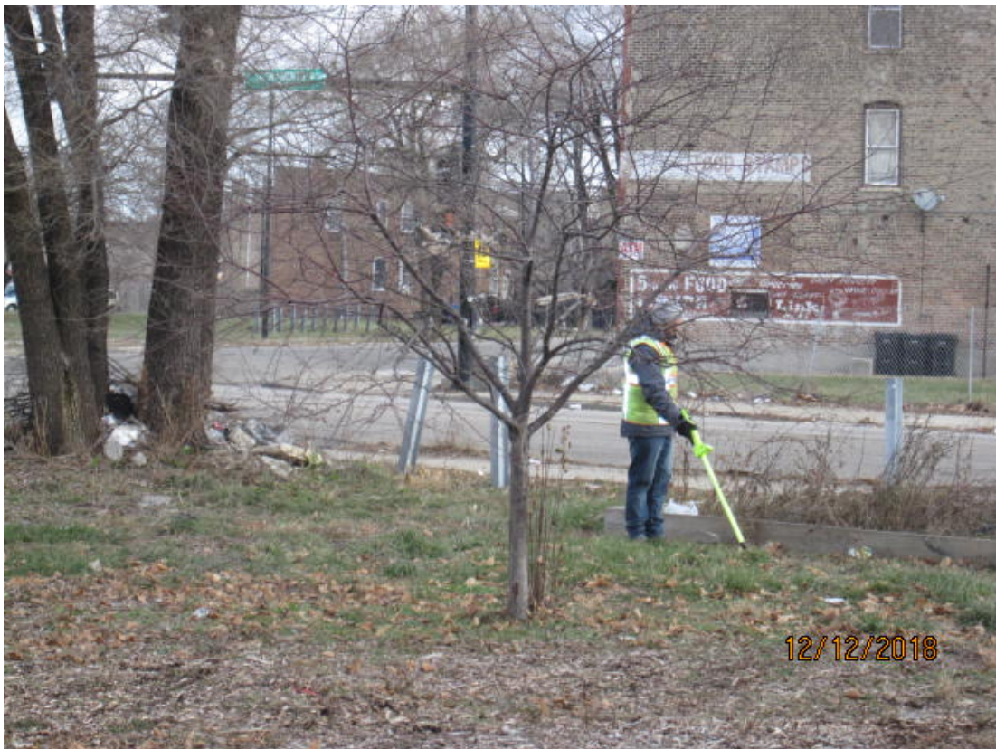
Photo 2: Electromagnetic (EM) survey activities (typical).
