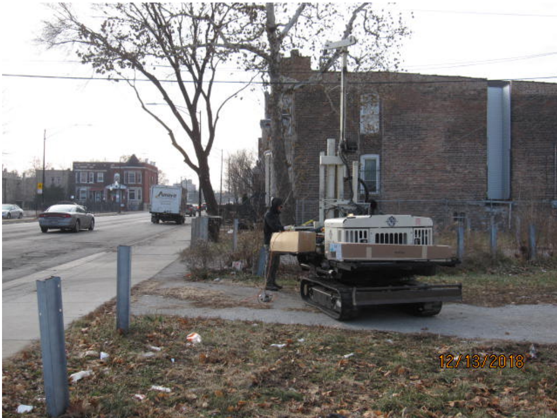
Photo 6: Advancement of soil boring SB-4.
