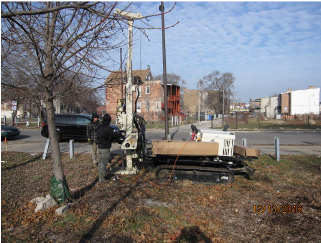
Photo 9: Advancement of soil boring SB-7.
