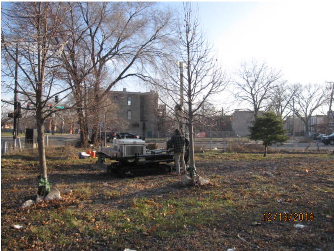
Photo 4: Advancement of soil boring SB-2.
