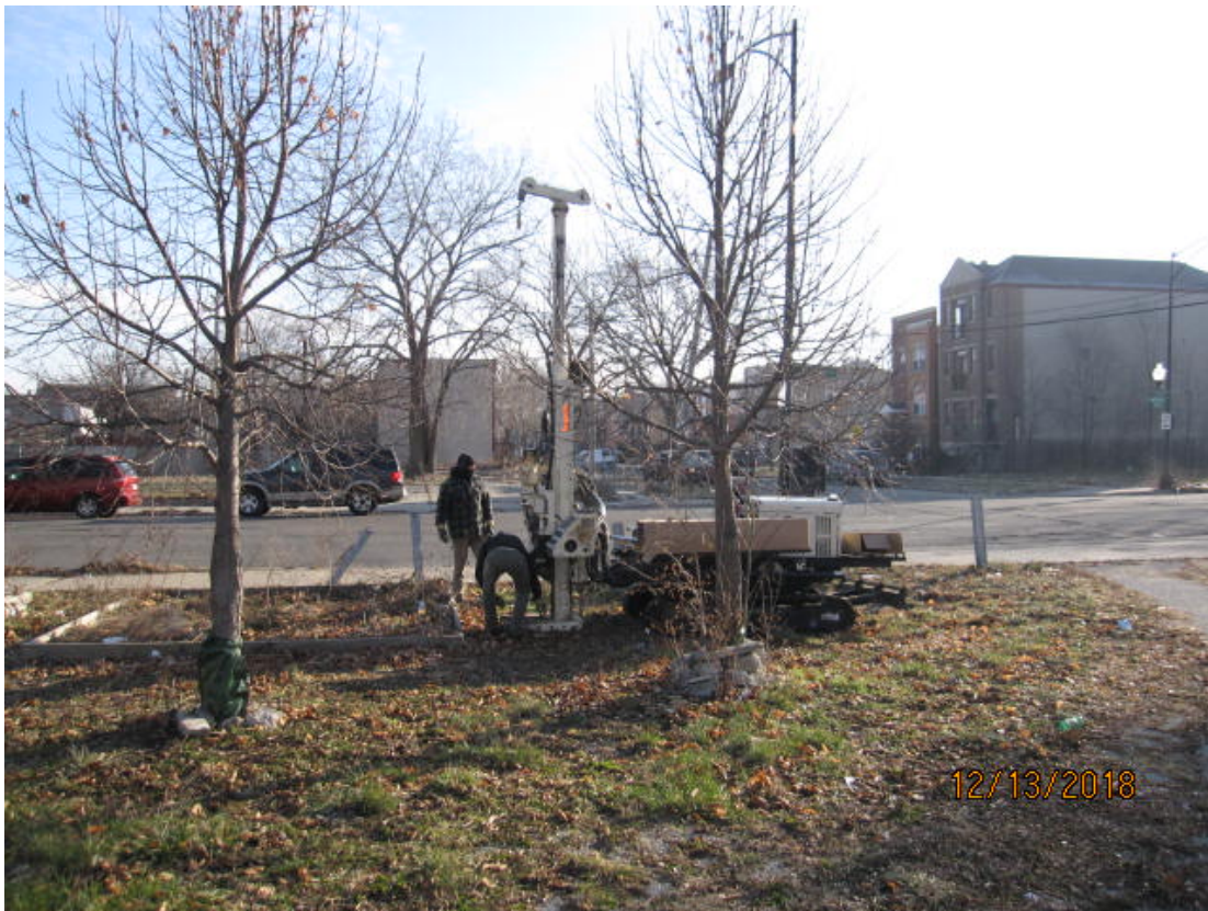
Photo 5: Advancement of soil boring SB-3.
