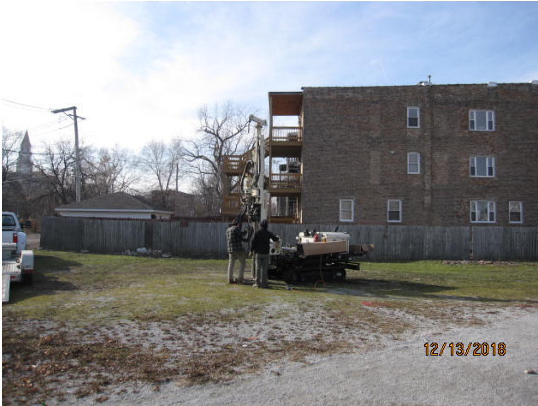
Photo 11: Advancement of soil boring SB-9.
