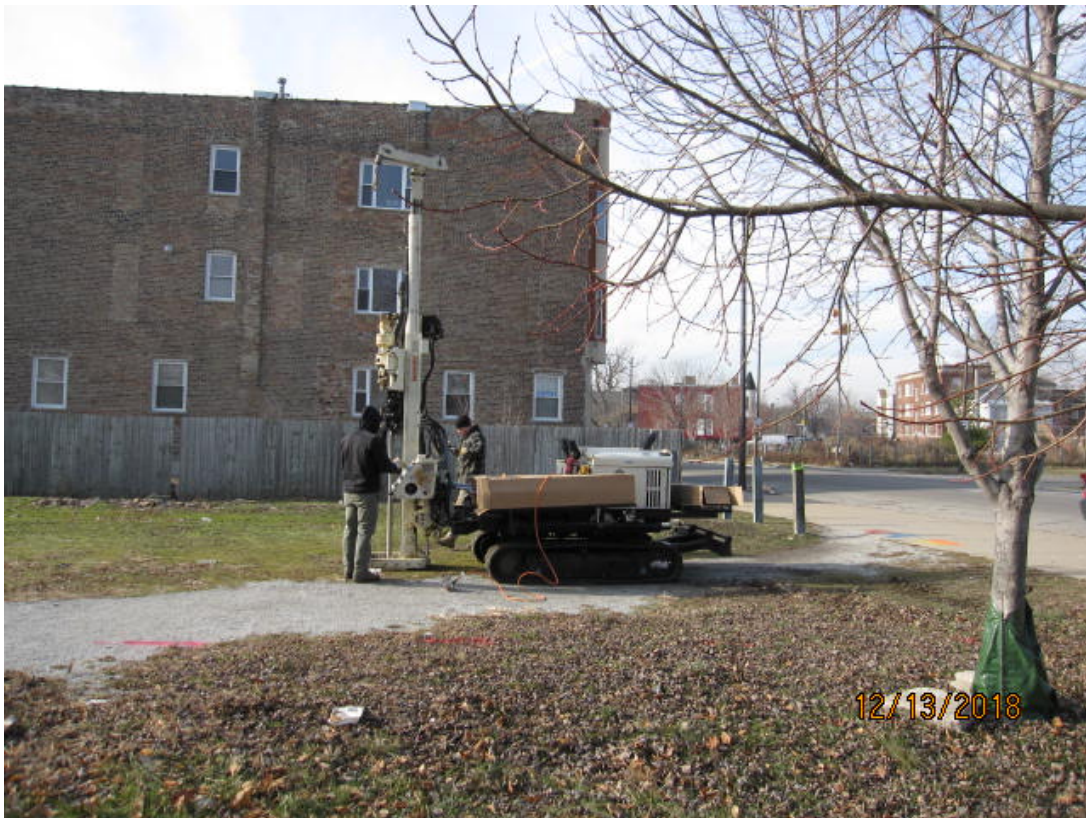
Photo 10: Advancement of soil boring SB-8.
