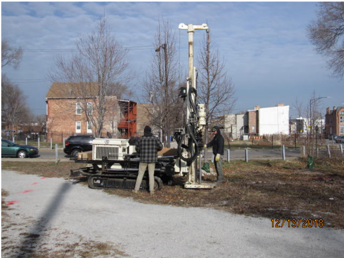
Photo 8: Advancement of soil boring SB-6.
