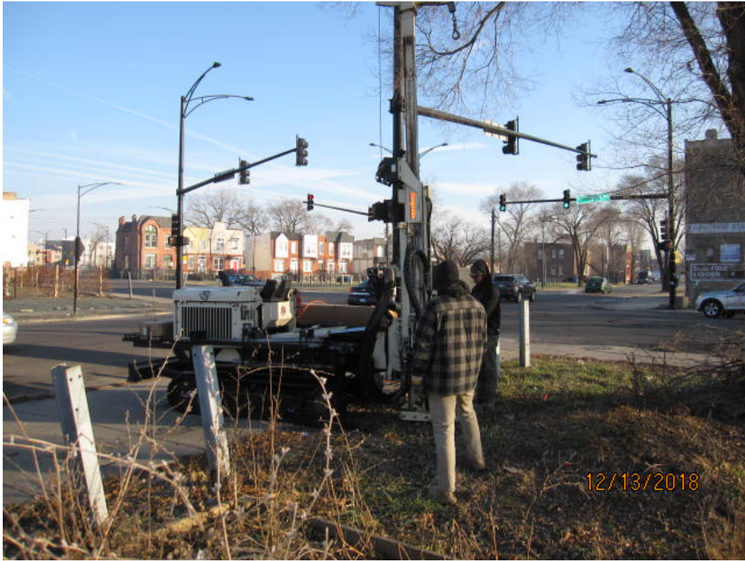
Photo 3: Advancement of soil boring SB-1.
