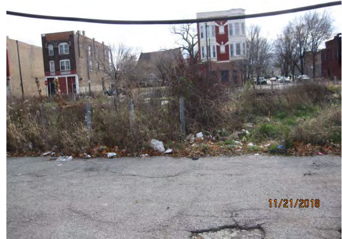
Photo 2: Rear view of 3024-40 W. Fifth Ave. looking southeast from the northern adjacent alleyway.
