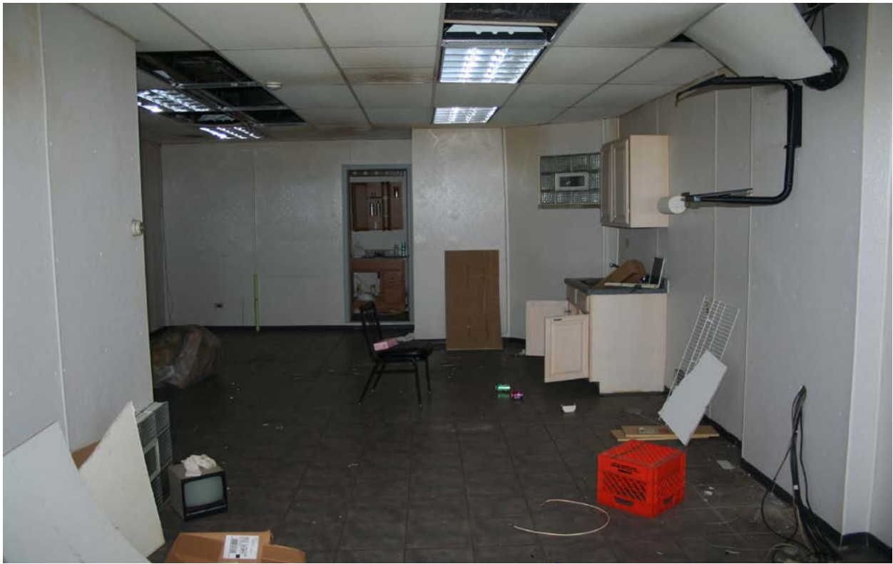
Photo 8: 2713 W. Division interior
