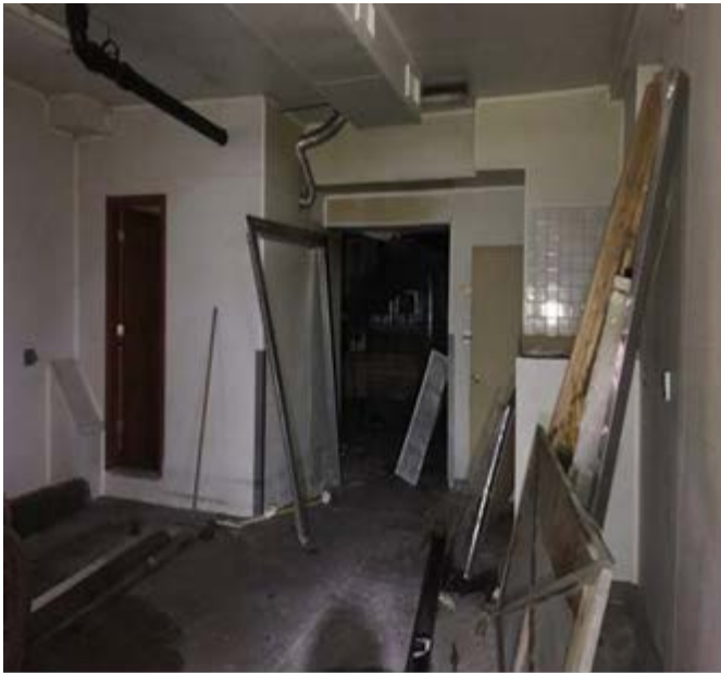
Photo 10: Interior lower level
