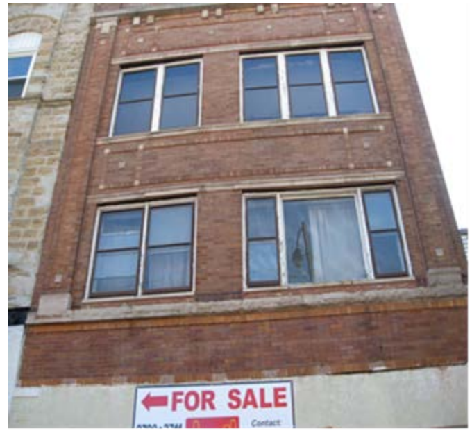
Photo 5: 2715 W. Division exterior
