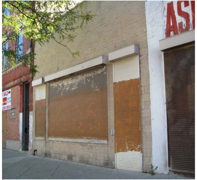
Photo 3: 2711 W. Division exterior
