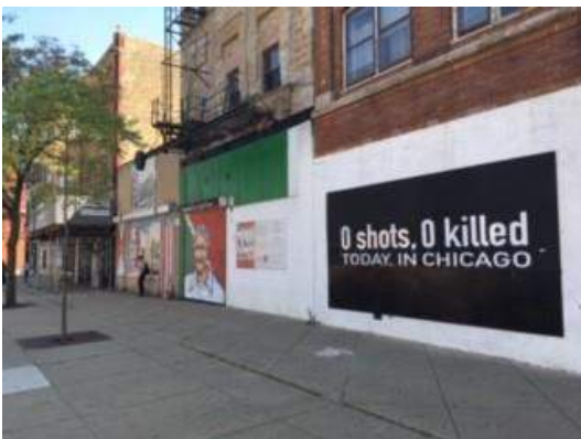
Photo 3: Subject site north facade, looking southeast from sidewalk
