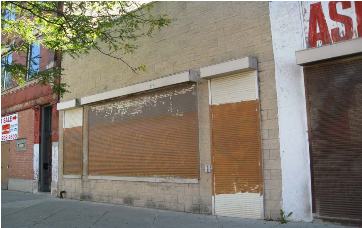
Photo 3: 2711 W. Division exterior
