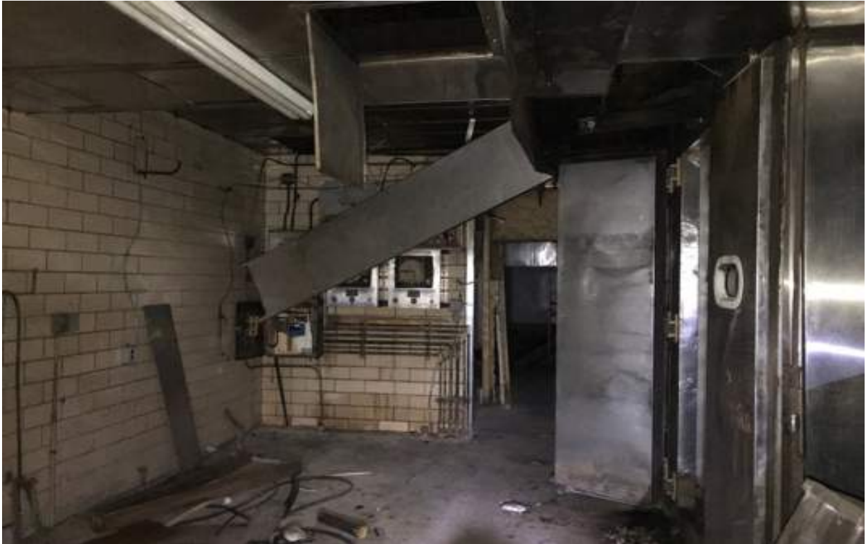
Photo 11: Basement interior view
