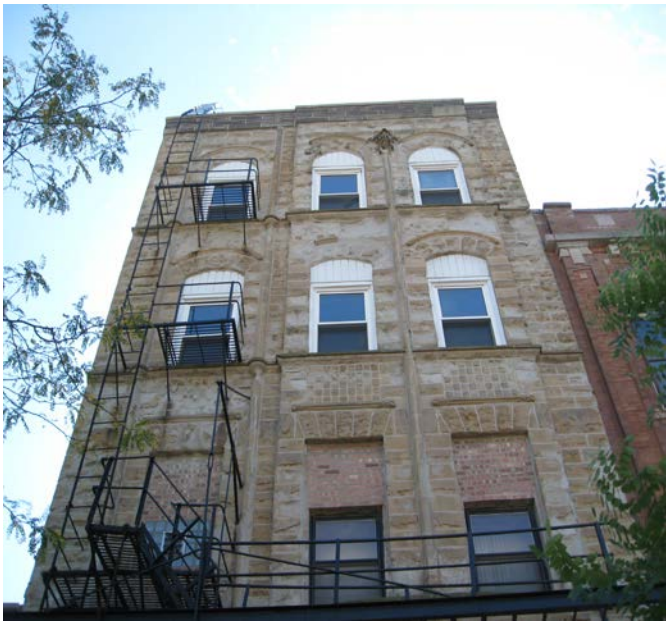
Photo 4: 2713 W. Division exterior
