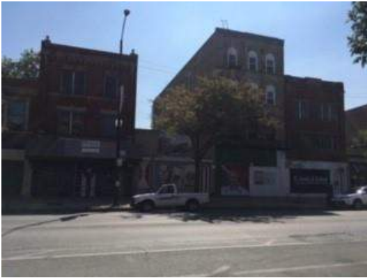
Photo 1: Subject site, looking south from across Division St.
