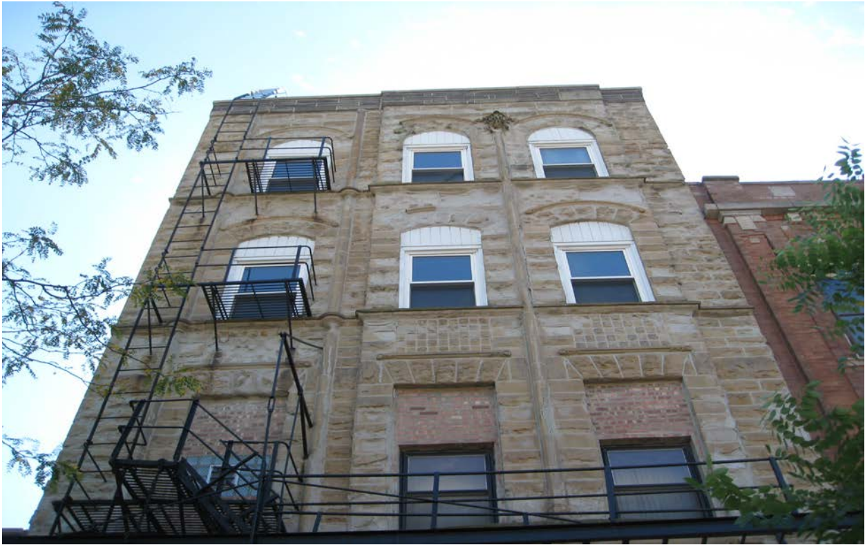
Photo 4: 2713 W. Division exterior
