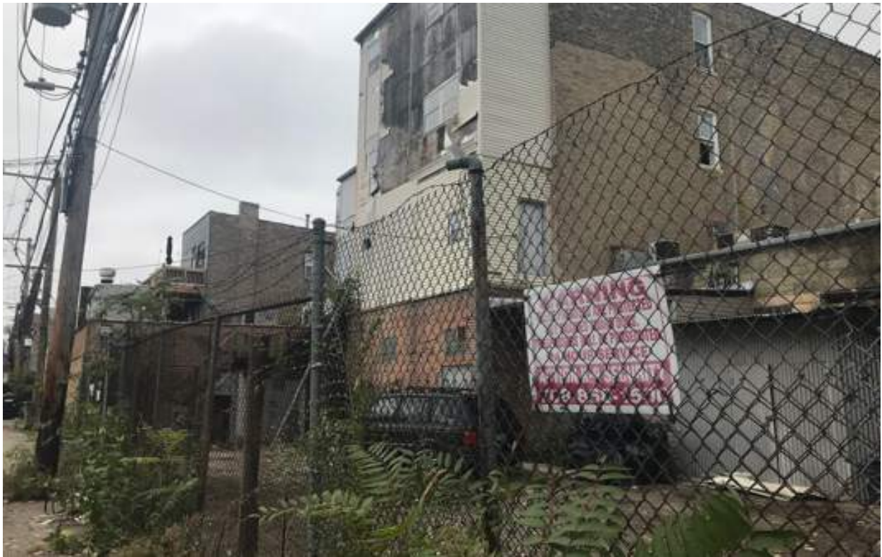
Photo 12: Rear of property
