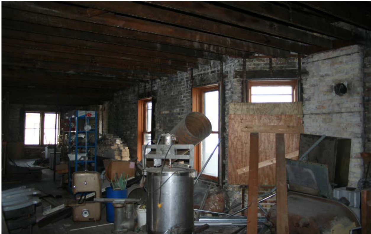
Photo 6: 2709 W. Division interior
