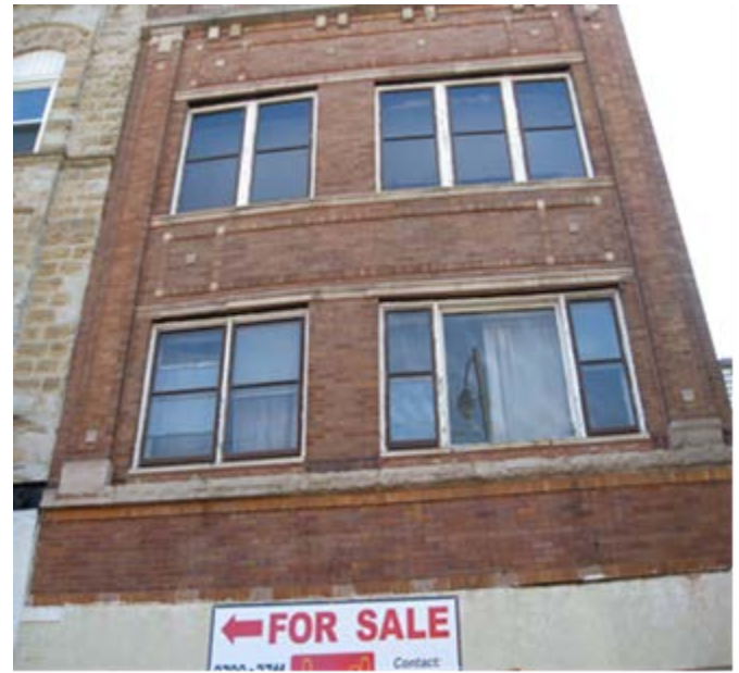
Photo 5: 2715 W. Division exterior
