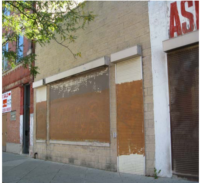
Photo 3: 2711 W. Division exterior
