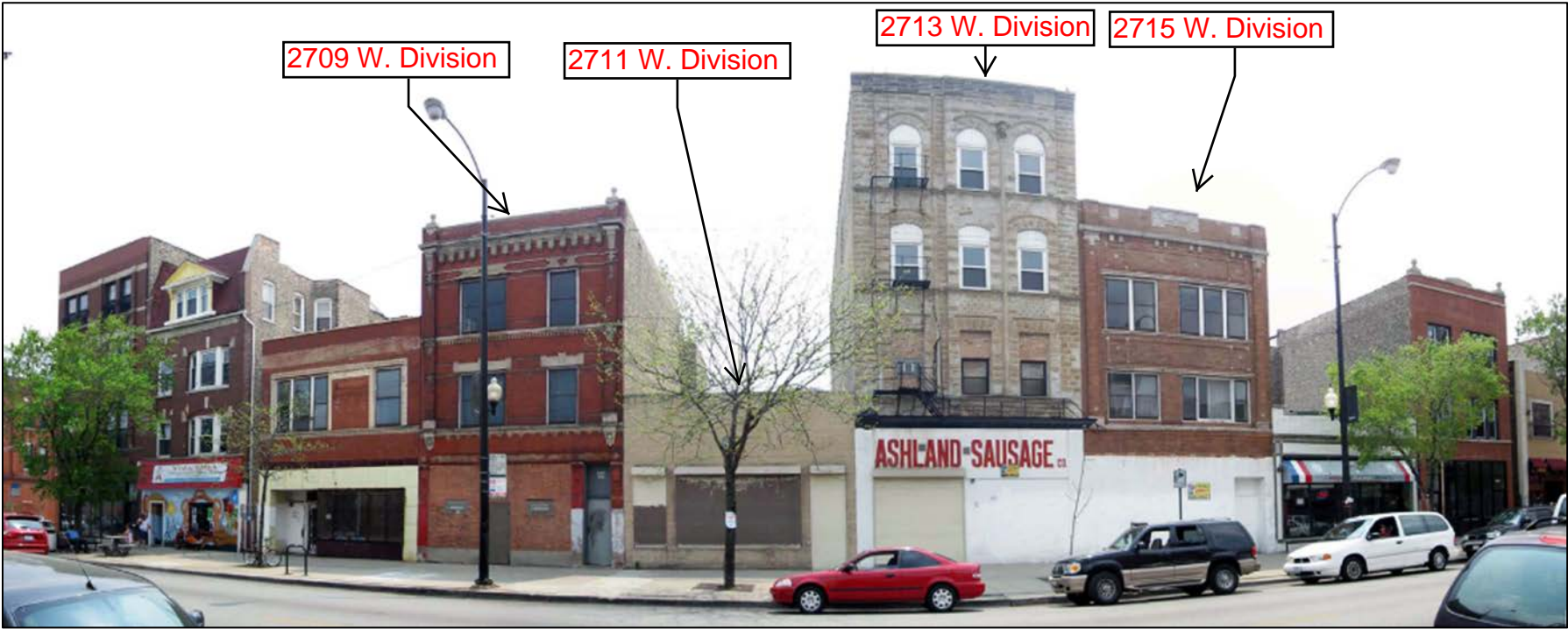
Photo 1: Project property photo of the four interconnected buildings
