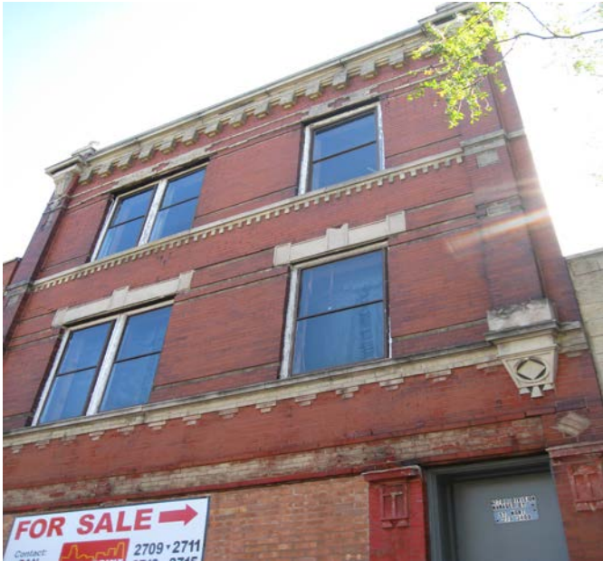
Photo 2: 2709 W. Division exterior
