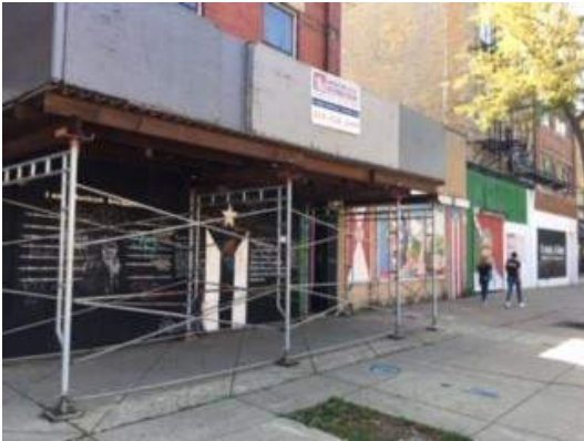
Photo 2: Subject site north facade, looking southwest from sidewalk
