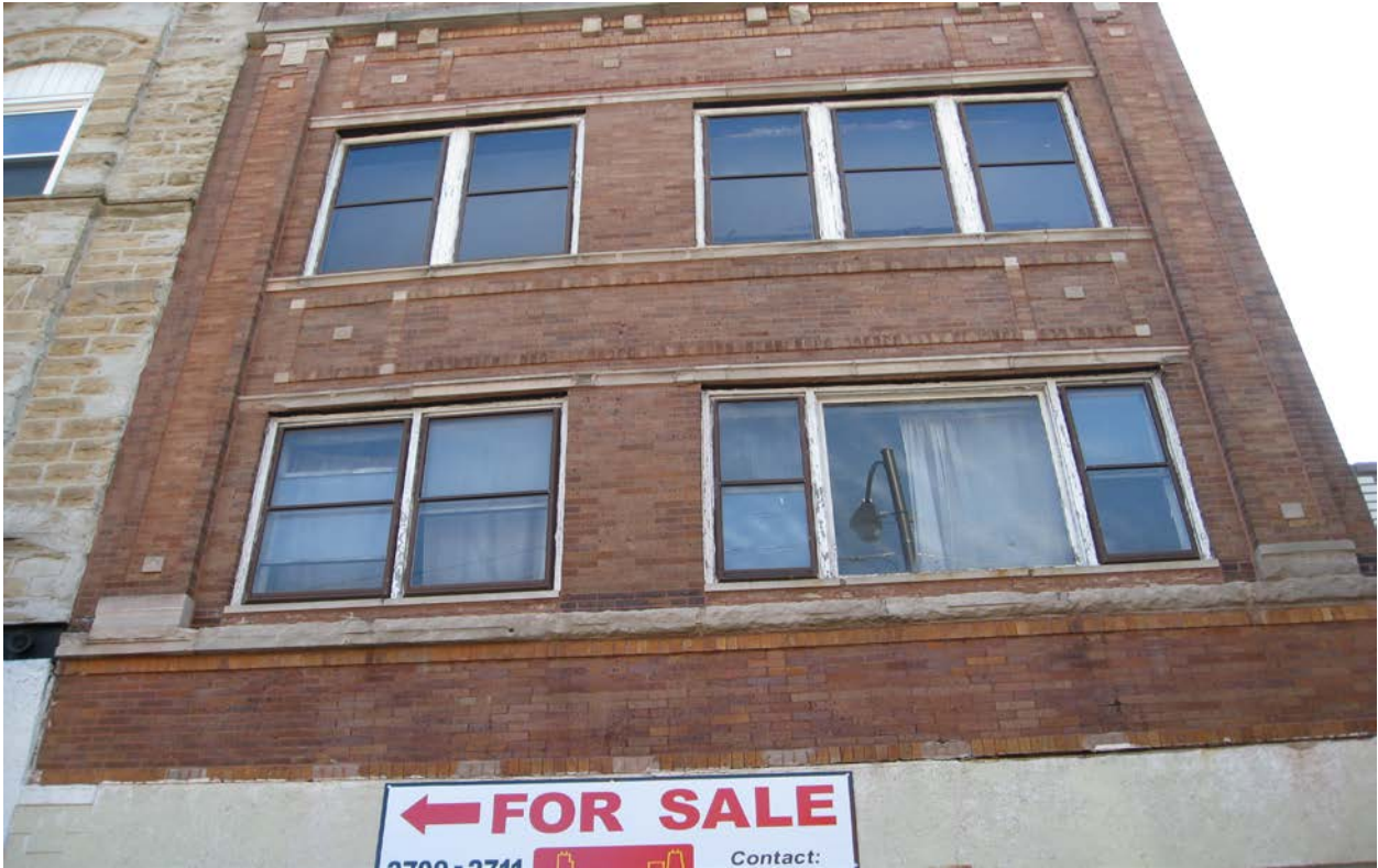
Photo 5: 2715 W. Division exterior
