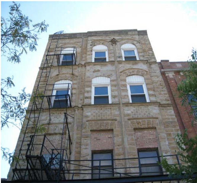
Photo 4: 2713 W. Division exterior
