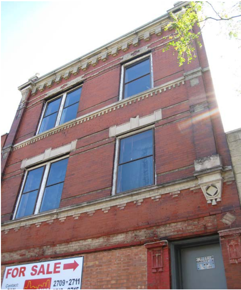
Photo 2: 2709 W. Division exterior
