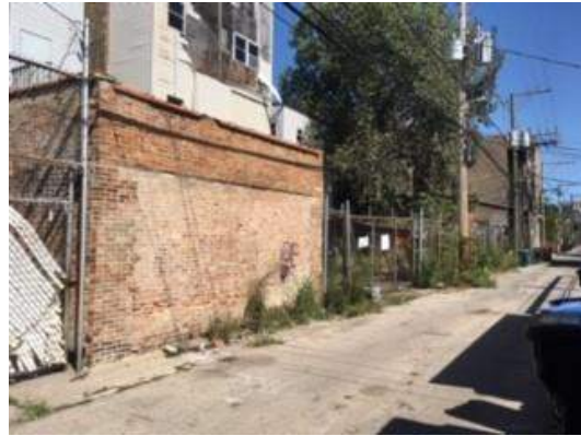
Photo 4: Subject site rear, looking northeast from alley
