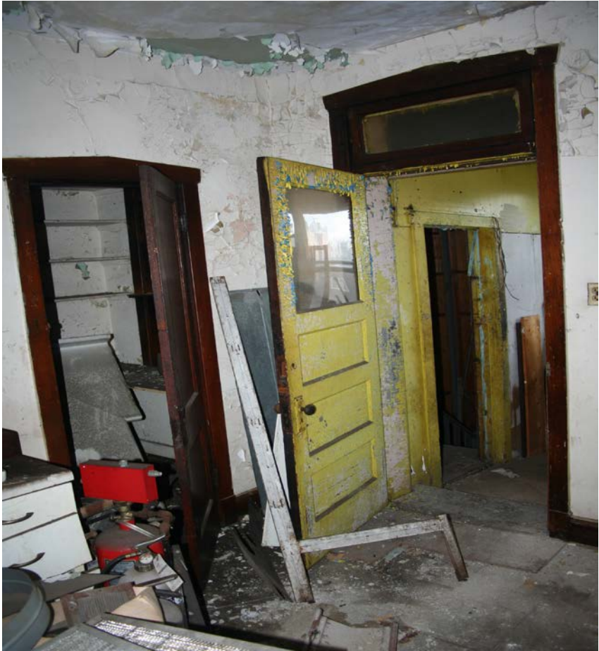
Photo 9: 2715 W. Division interior
