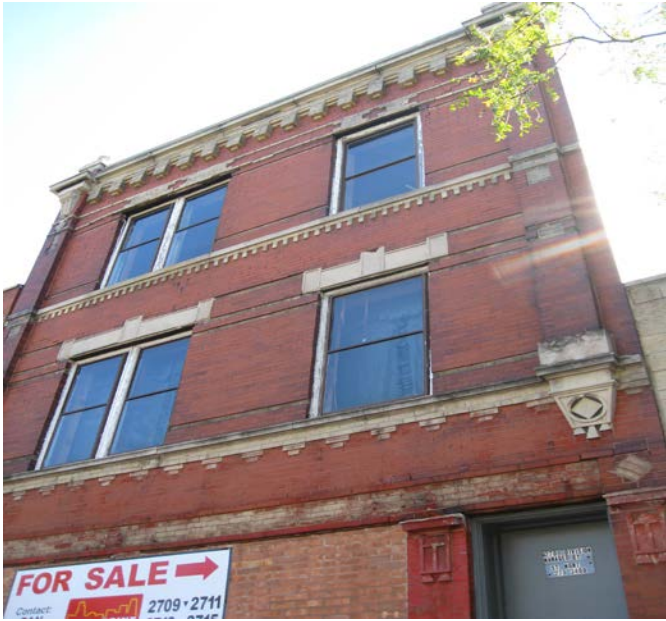
Photo 2: 2709 W. Division exterior
