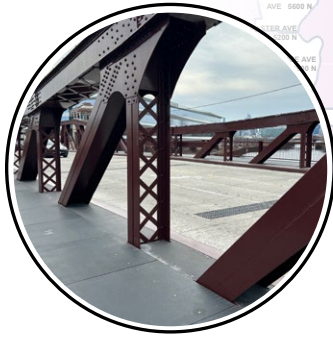
BUCKTOWN Webster Bridge Webster St. from Ashland to Dominick
