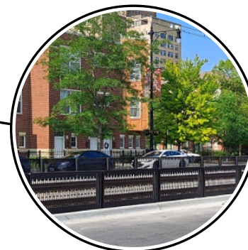
SOUTH SHORE 71st Street Streetscape 71st/Stony Island
