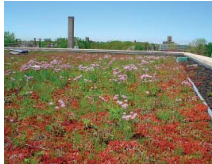
Figure 3-LA6 . Example of Green Roof Vegetation
