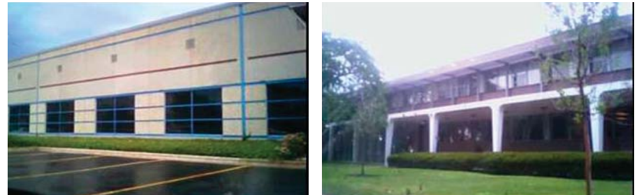
Figure 3-AR4. Bradley Business Center Figure 3-AR5. Wrightwood\Bodine Building
