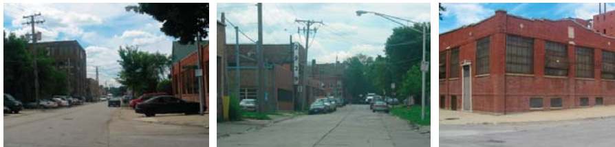
Figure 3-UD18. Existing stock of industrial buildings
