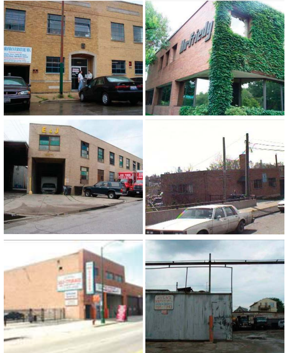
Figure 3-AR1: Existing Buildings in Corridor
