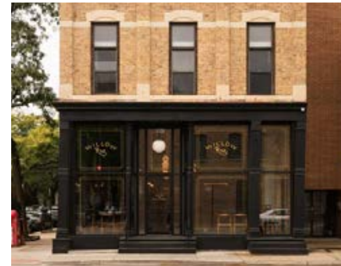
Clear and visible main storefront entrance.
