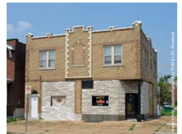
X Not Recommended: Using materials that don't complement the architectural style and infilling the existing window openings.
