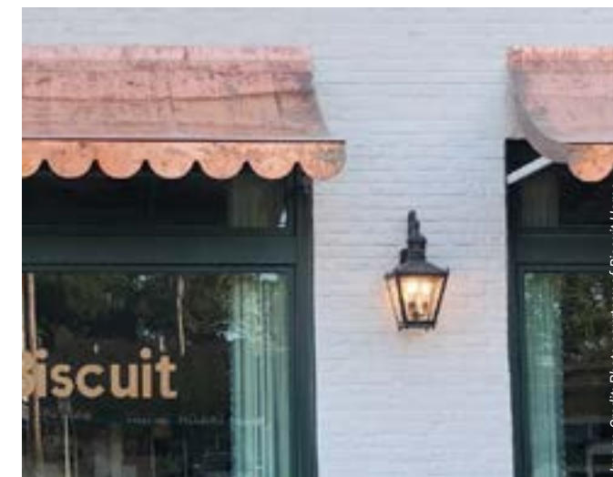
Sconce light along storefront facade.
