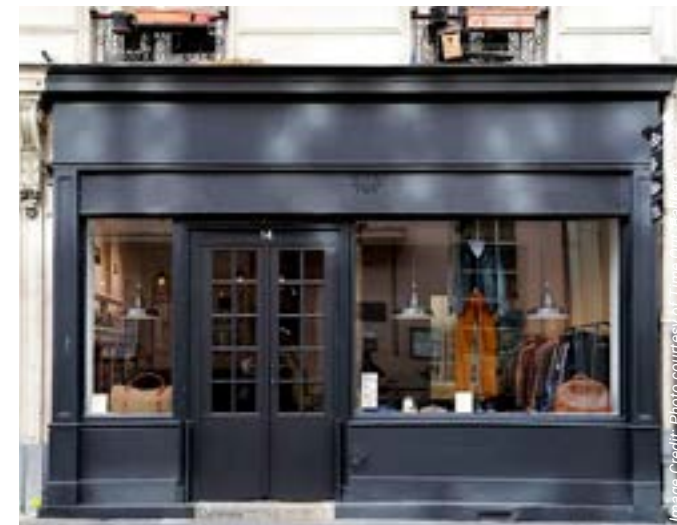
Double doors consisting of wood and small glass panels.
