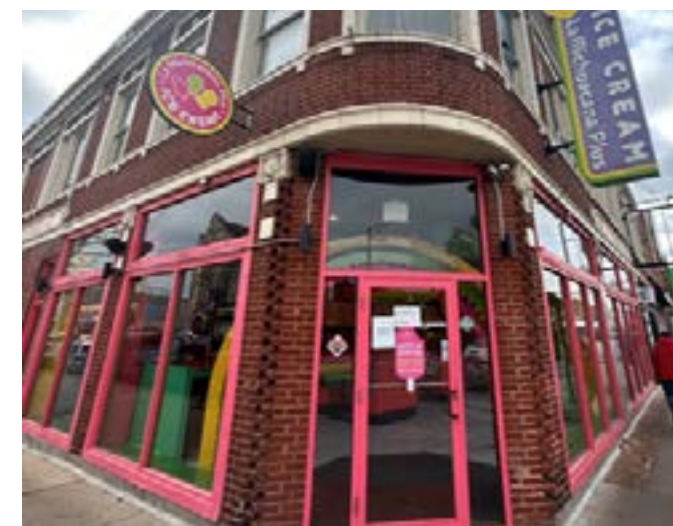
Angled entry for a corner store allows convenient access from both directions.
