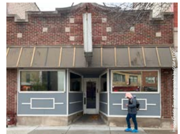
X Not Recommended: Deeply recessed and dark entries that create an unwelcoming space.
