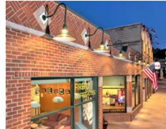
Goose-neck lighting to illuminate the sidewalk.
