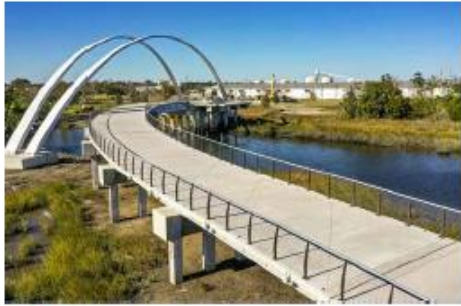
Noisette Creek Ped. Bridge - North Charleston, SC
