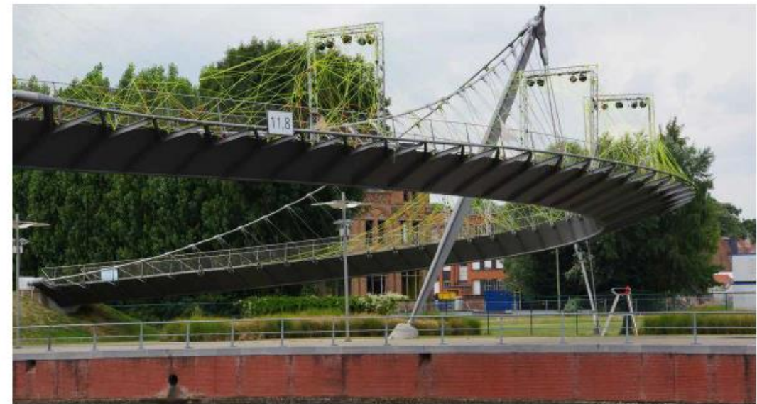
College Footbridge - Belgium
