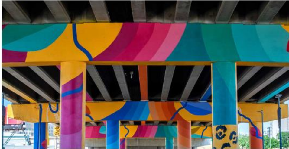
Sun Valley Viaduct - Denver, CO
