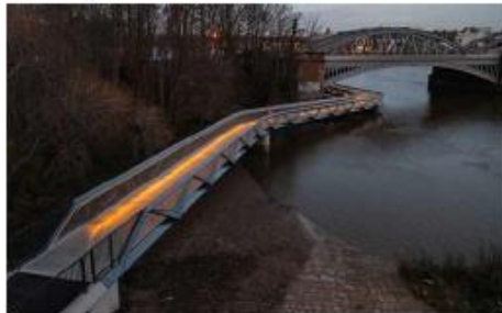
Dukes Meadow Footbridge - London, United Kingdom
