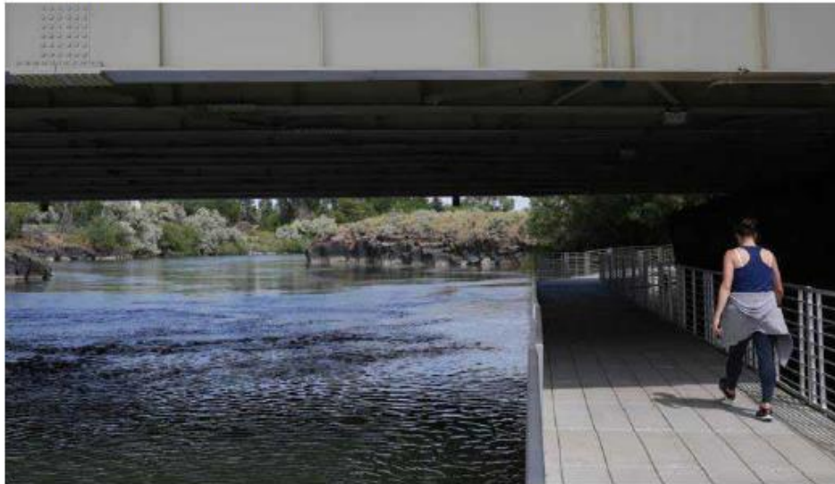
Floating bridge in Idaho Falls, ID
