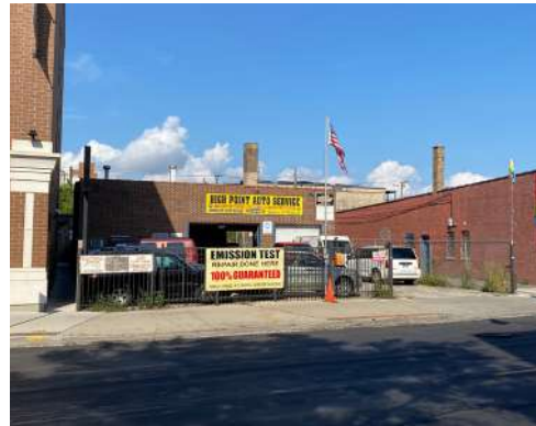
E High Point Auto Service – 4922 N Clark Use: Vehicle service with outdoor storage of vehicles
