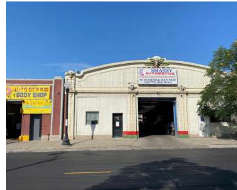
G Smashy Automotive – 5006 N Clark Curb cuts on Clark Street Insufficient storefront transparency
