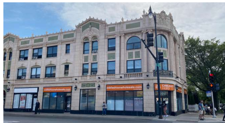
Issel Building (c. 1929) 4532-4558 N Clark St – Landmark
