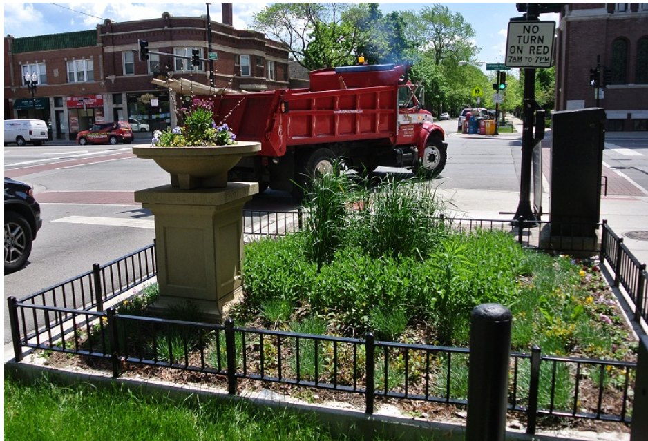
Photo: An example of a landscaped planter urn at the bump-out constructed on the corner of Irving Park Road and Leavitt Street as part of the first phase of the Irving Park Road Streetscape project.
