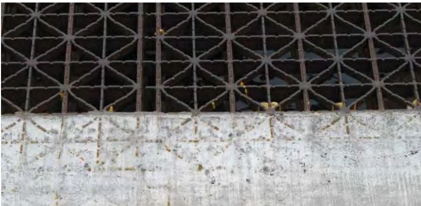
Open grate bridge treated with concrete infill on Van Buren Street
