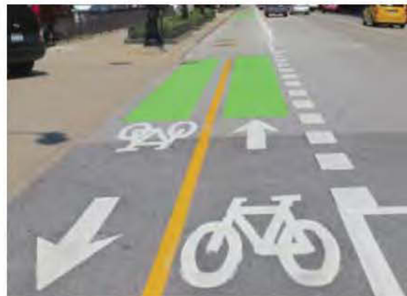
Green pavement at driveways
