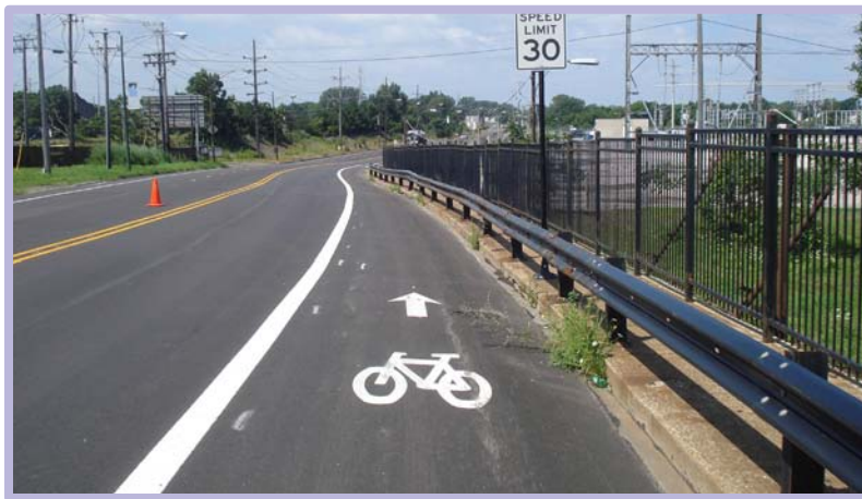
100th St. - Looking west from bridge over Calumet River
