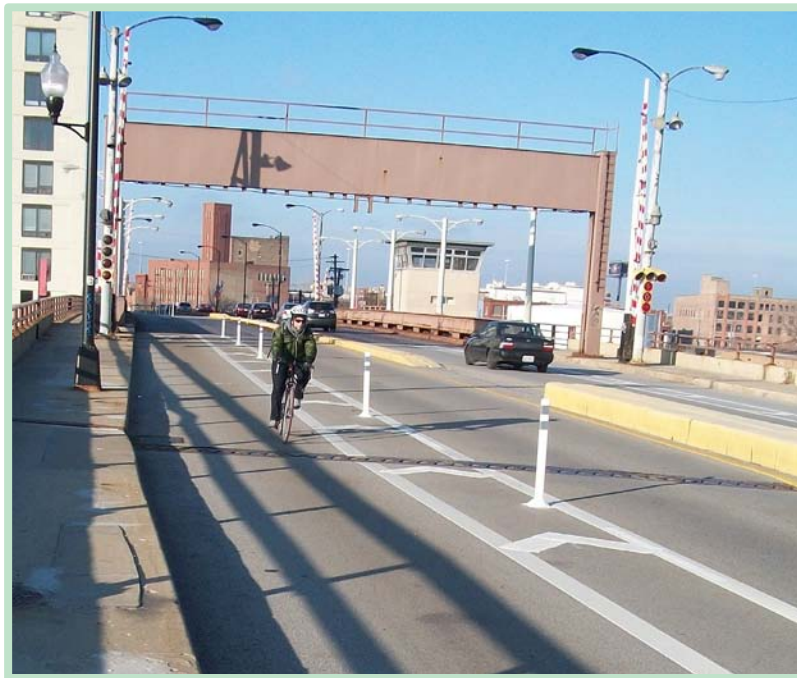
18th St. Bridge - Looking west
