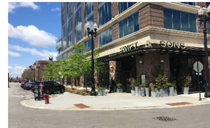
Curb Extensions / ADA Upgrades
