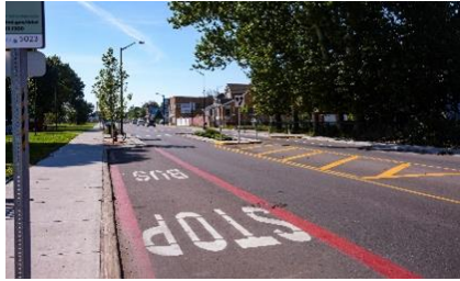
Road Resurfacing & Pavement Markings
