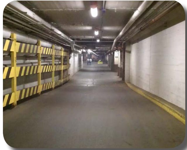
Existing below-grade passageway could be upgraded for passengers using converted mail platforms
