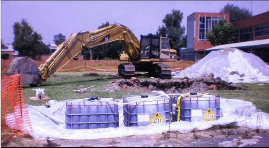
Photo: ISCO Soil Mixing
