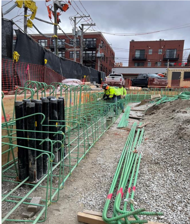
Forming Grade Beams at Damen
