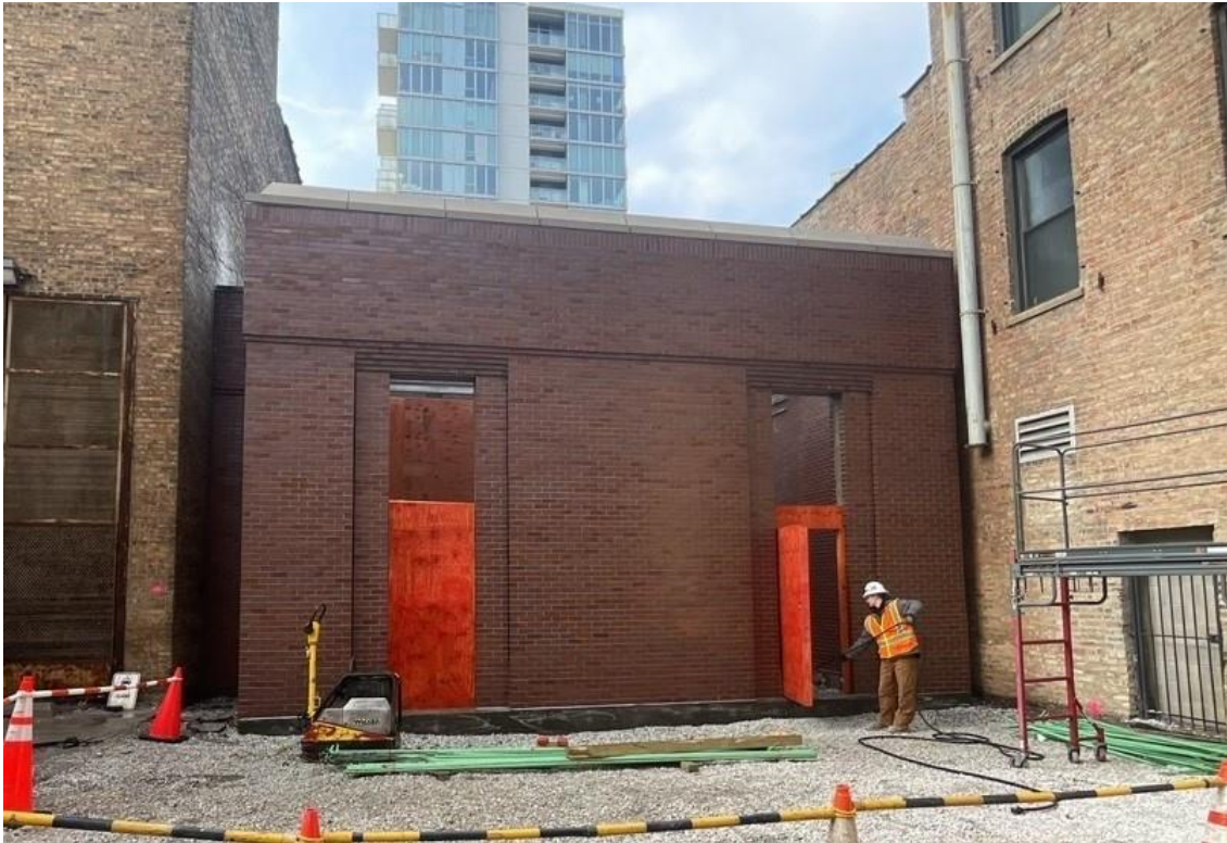
Completed East Wall at Haymarket
