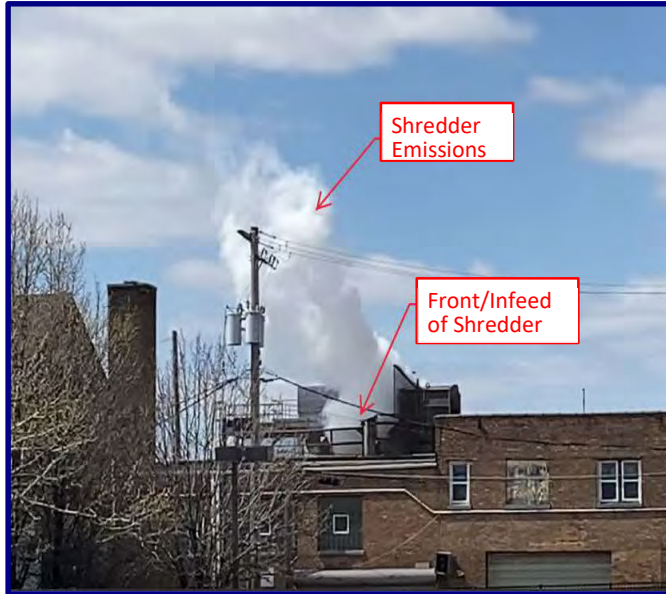
Figure 2 – Typical Uncontrolled Exhaust from Front/Infeed of the Hammermill Shredder at SIMS South Paulina
